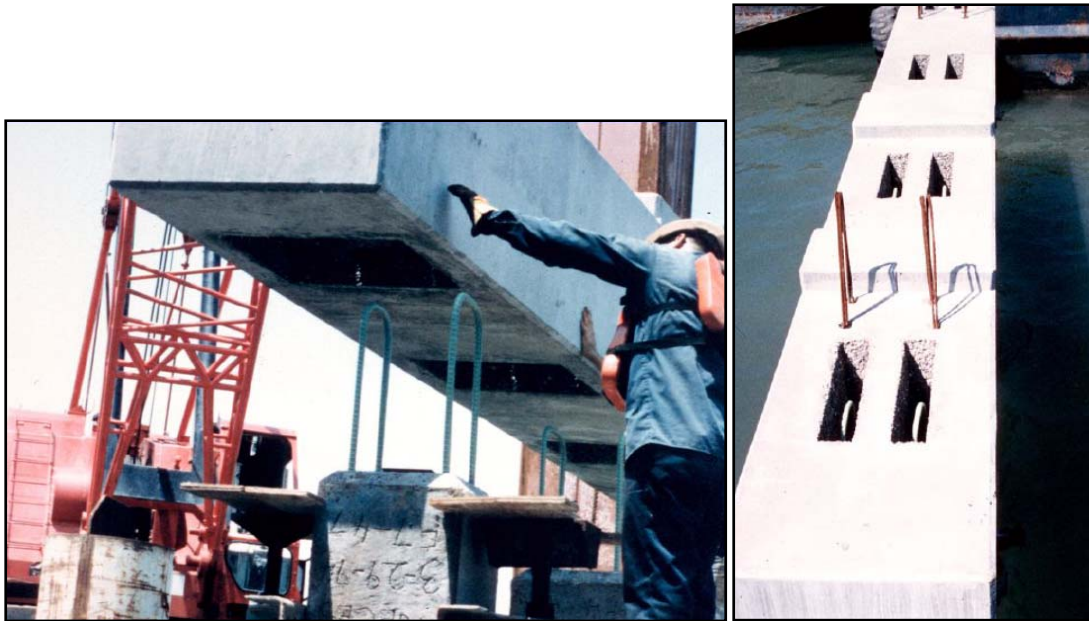
Figure 9 – Grouted Pocket Connection (14)
