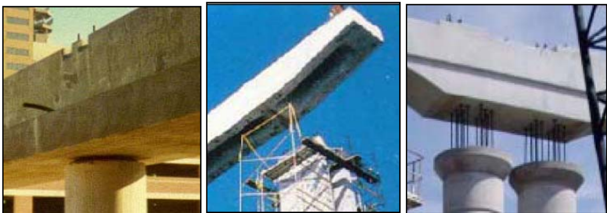
Figure 8 – Pier Cap to Column connections: Bolted connection (13) (left), connection by splice sleeves (5) (middle), grouted duct connection (14) (right)
