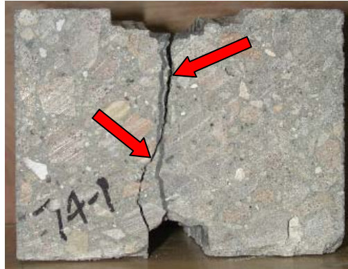
Figure 4.2.2 Example of a concrete failure.
