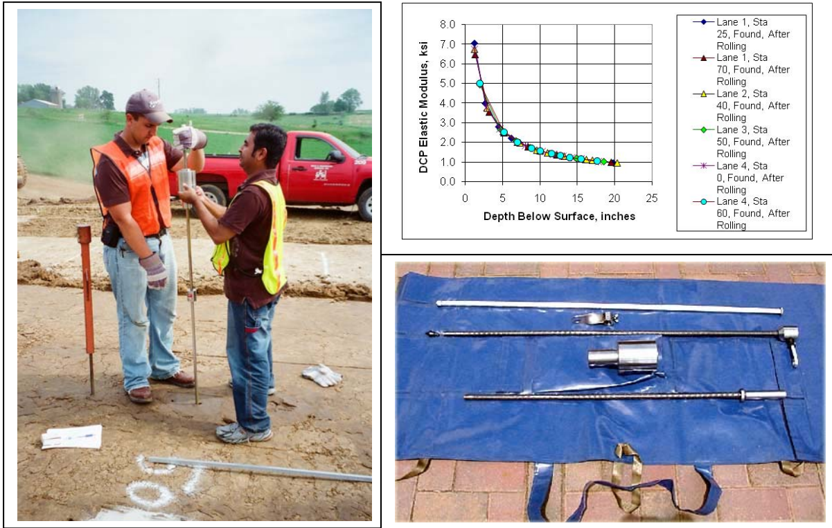
Figure 40. DCP Test and Equipment, and Example of Calculated Resilient Modulus from the Penetration Rate with Depth
