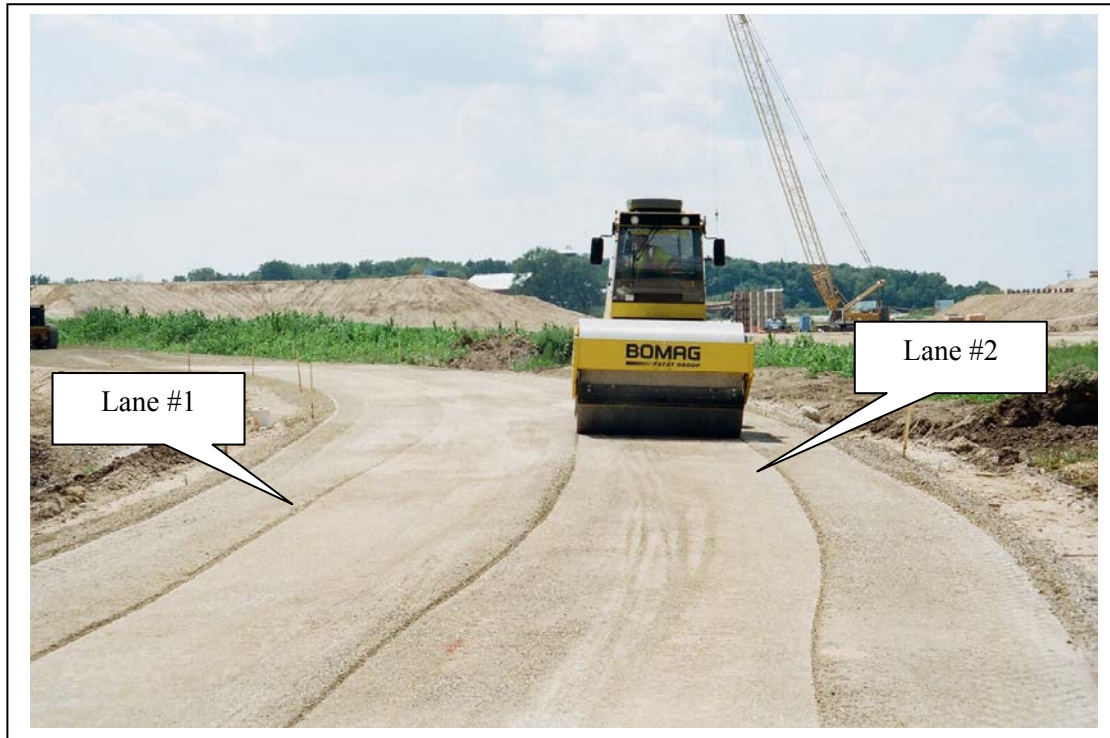
Figure 33. Jefferson STH 18 Project; Crushed Aggregate Base, Both Lanes Included in Project
