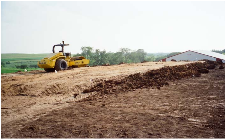
Figure 26. Highland STH 80 Project; High Plasticity Clay Embankment Test Area
