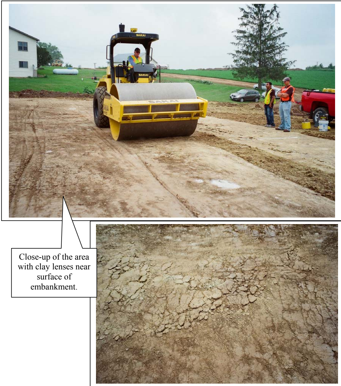
Figure 61. Condition of the Surface of the High Plasticity Clay Embankment during the Compaction Process (Highland Project)
