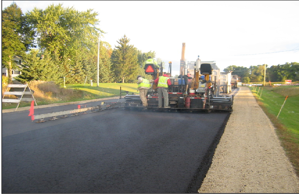
Figure 34. Eden USH 45 Project; HMA Paving
