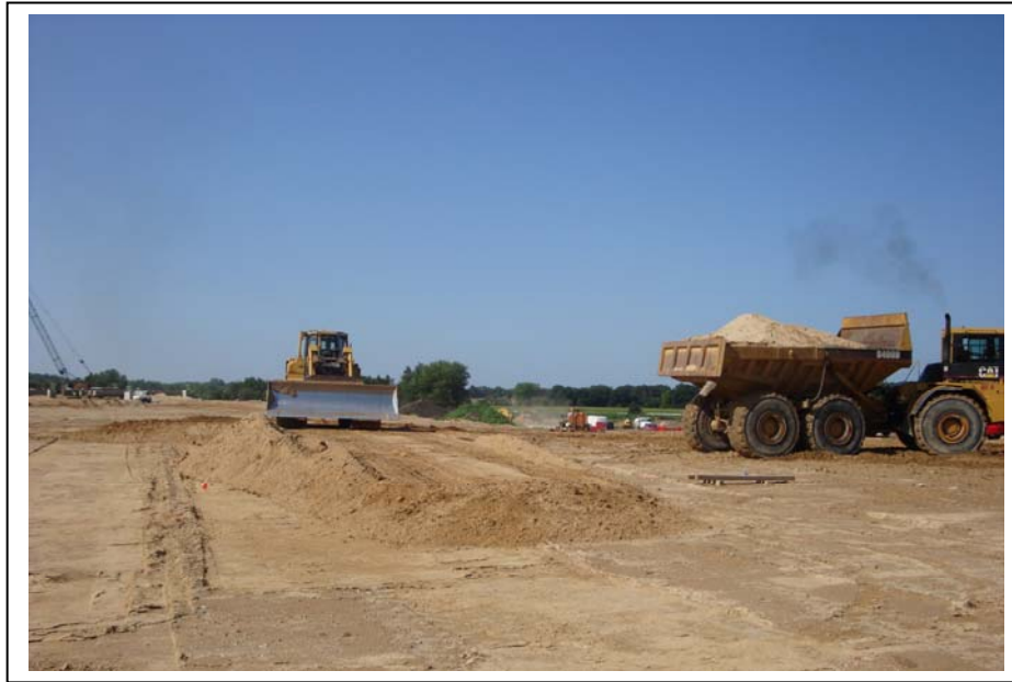
Figure 29. Jefferson STH 18 Project; Placement and Spreading of the Embankment Soils
