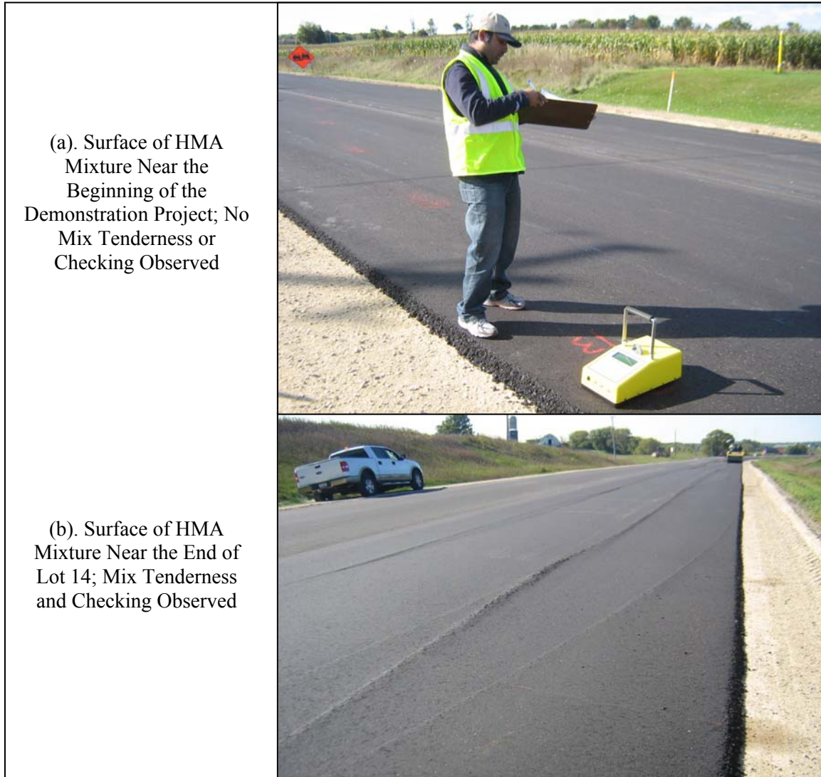
Figure 77. Surface of HMA 19-mm Lift After IC Rolling
