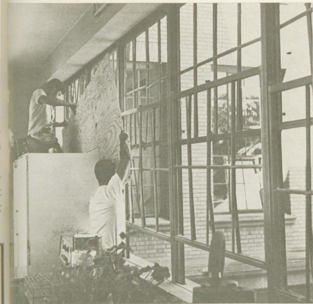
Above) Plywood is installed in the walkway between Old McArdle and S.M.I. Note how force of the blast bent window frames. (Below) Workers lift a manhole cover to inspect for gas leaks. Med center is in background.
