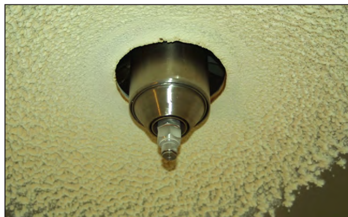
Deposits on top of dryer where wall temperatures are highest.
