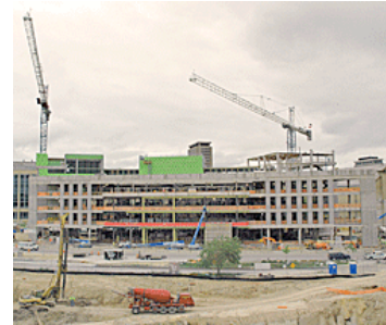
Wisconsin Institutes for Discovery building under construction. (large image)
