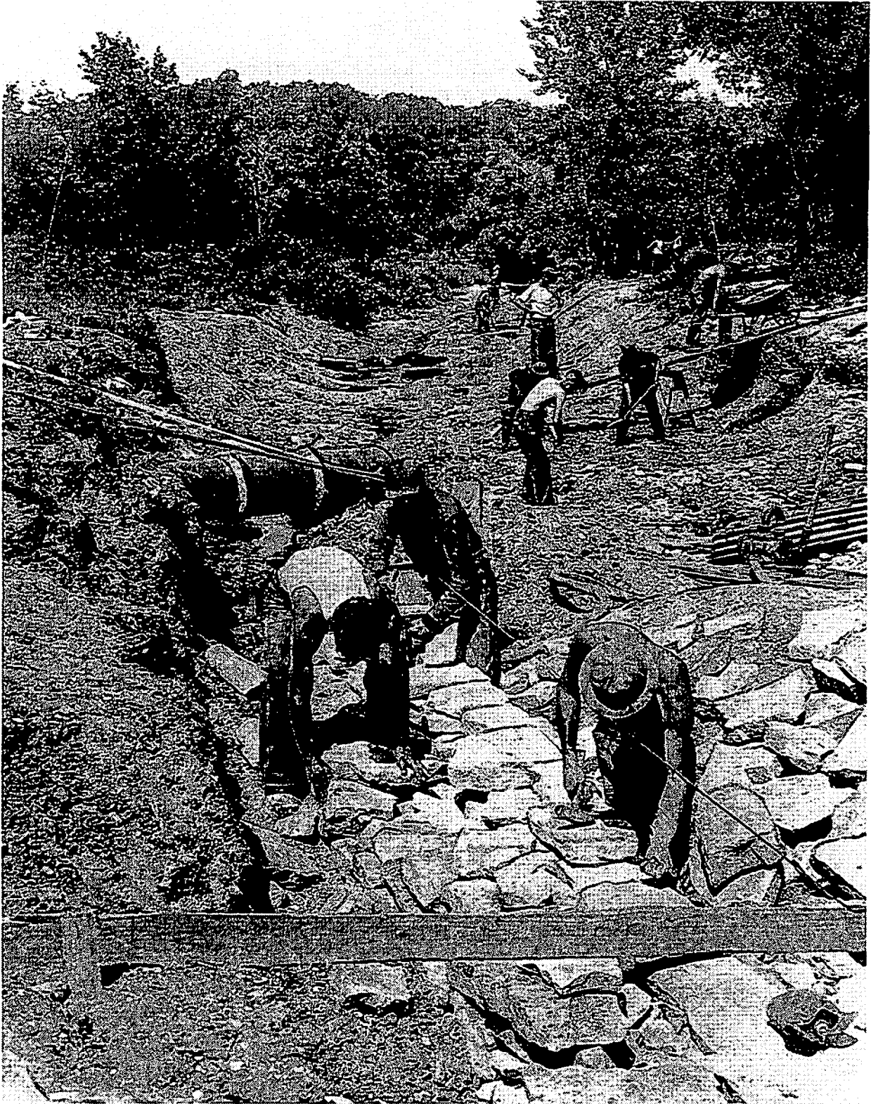
Milwaukee County Civilian Conservation Corps workers build revetments along the banks of Honey Creek in July 1933. Photograph courtesy of the Milwaukee Journal
