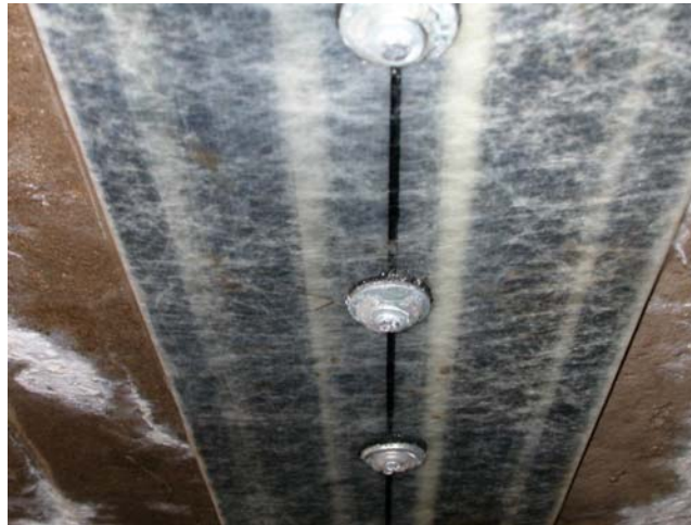
Figure 4.22. Properly installed ALH fasteners at the midspan
