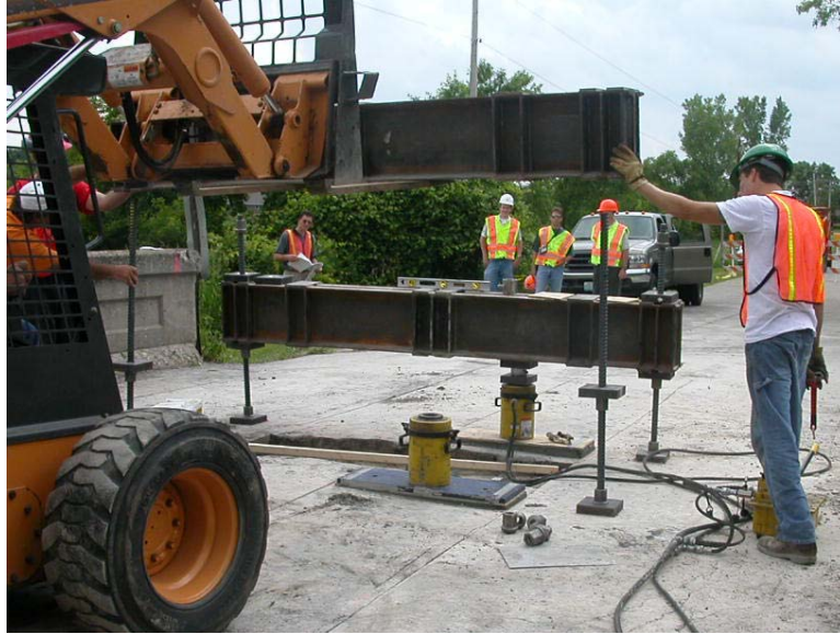
Figure 6.9. Placing the north reaction beam
