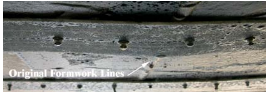
Figure 4.31. FRP strips fastened over original formwork lines
