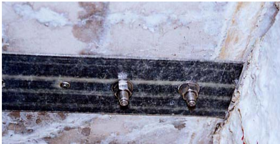
Figure 4.24. Installed end anchor next to the abutment
