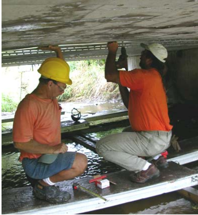
Figure 4.20. Pre-drilling into the concrete substrate at the midspan
