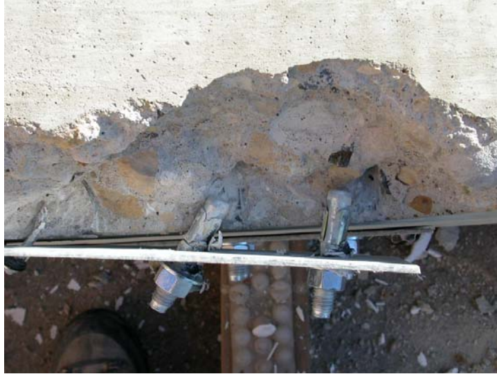
Figure 5.49. Final end-anchor pullout failure in beam FRP 3
