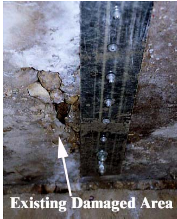
Figure 4.29. Relocated FRP strip near existing local damaged area
