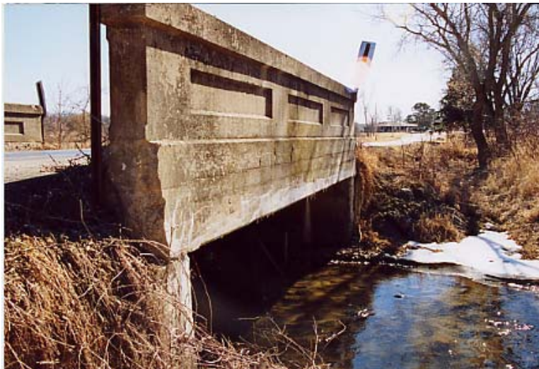
Figure 4.6. Depth of Creek under Bridge P-53-702
