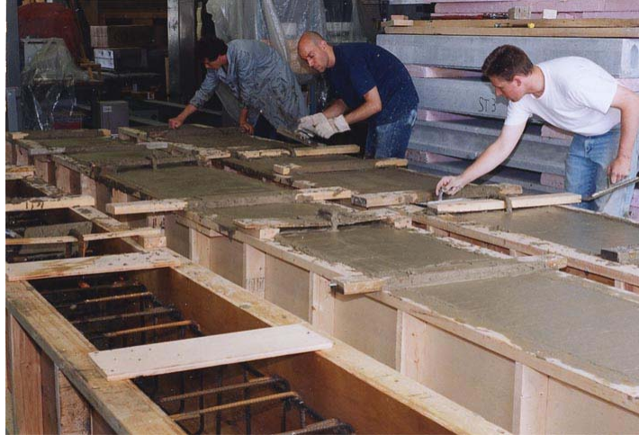
Figure 5.5. Finishing of the concrete
