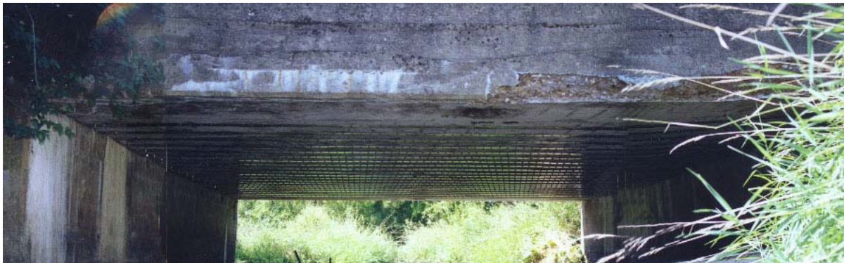
Figure 4.26. Bridge P-53-702 strengthened using MF-FRP system
