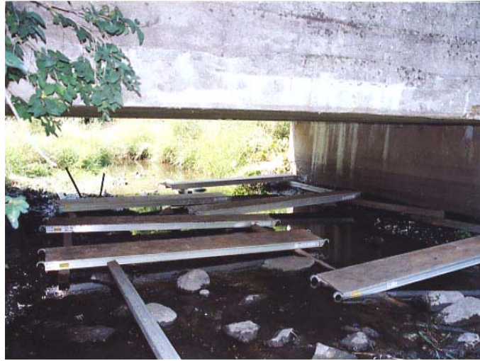
Figure 4.17. Working platform under the bridge
