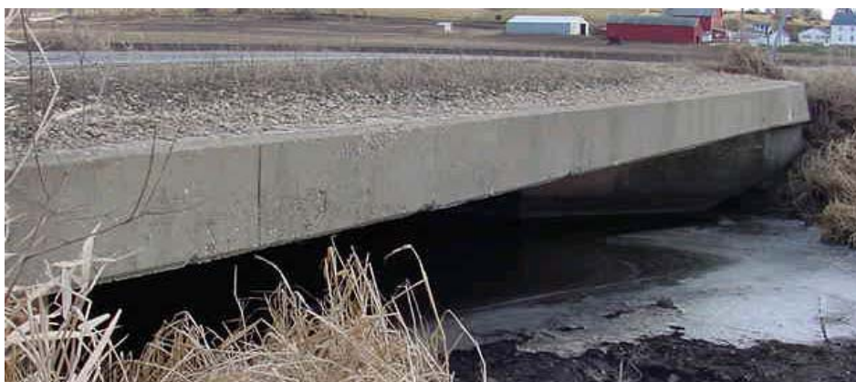
Figure 4.2. Slab of bridge B-13-518
