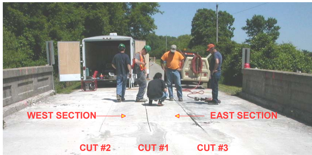
Figure 6.4. Test sections (looking north)
