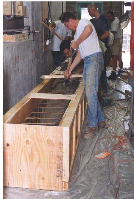
Figure 5.4. Concrete casting
