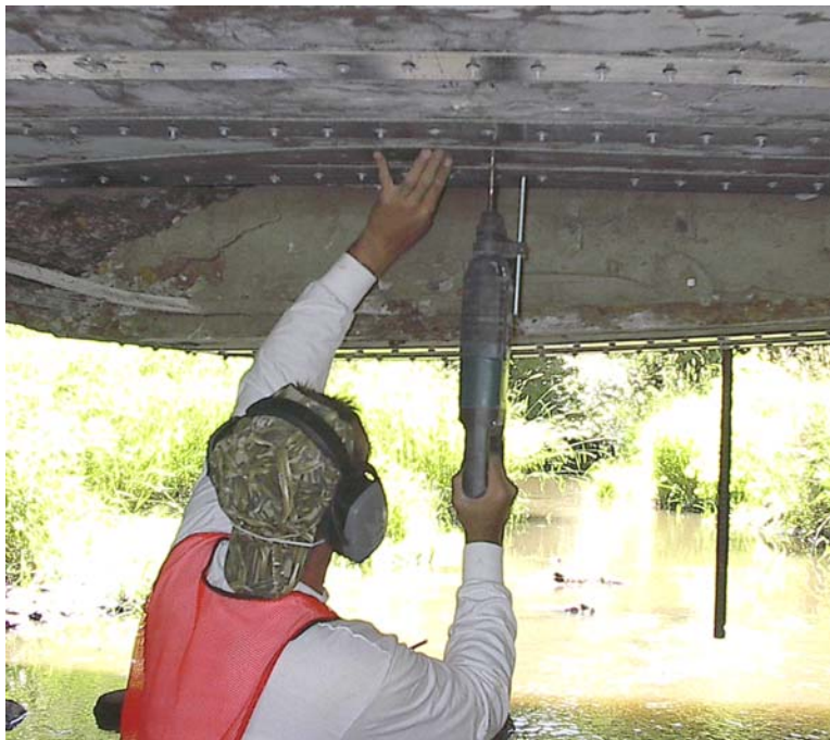
Figure 6.14. Pre-drilling the concrete prior to fastening the first additional strip
