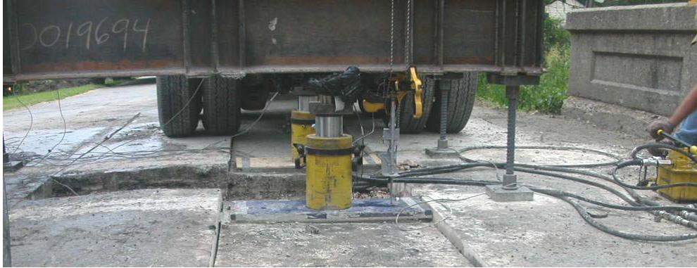
Figure 6.13. Testing the west section
