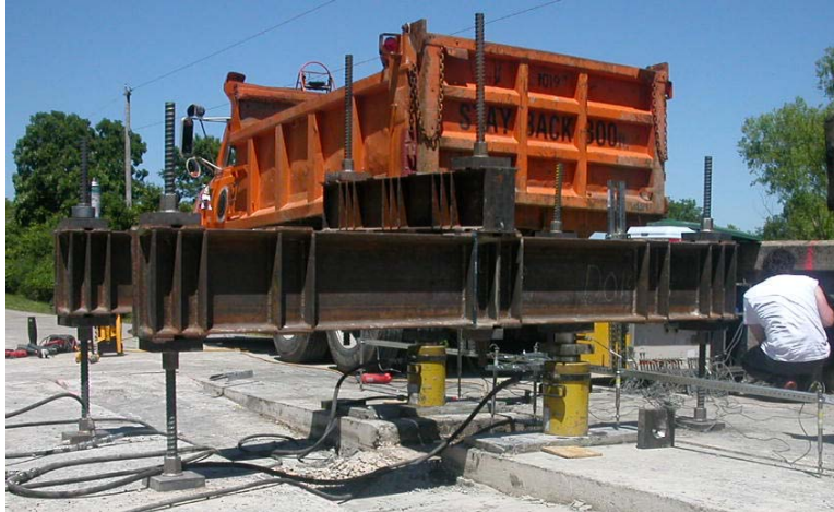
Figure 6.17. Testing the east section
