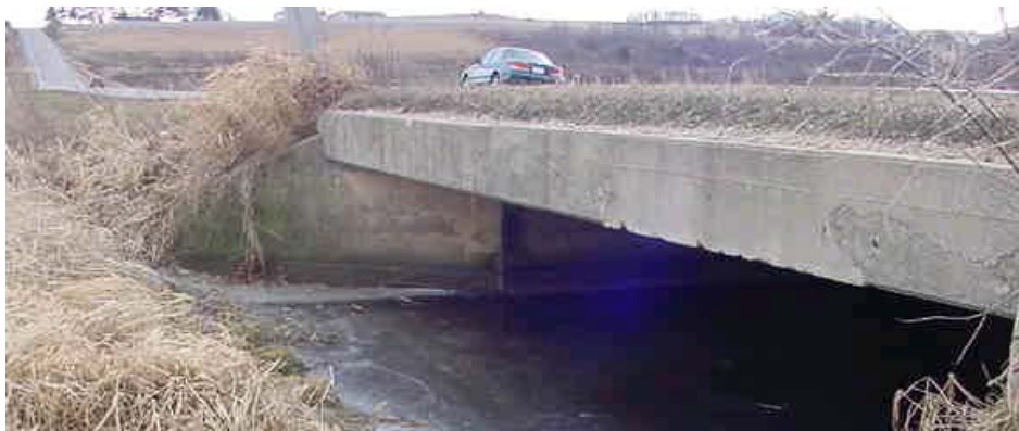
Figure 4.1. View of Bridge B-13-518
