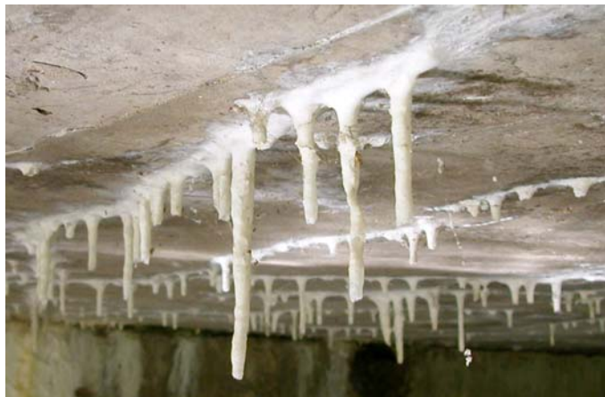
Figure 4.18. Soft calcium stalactites seen on the concrete substrate
