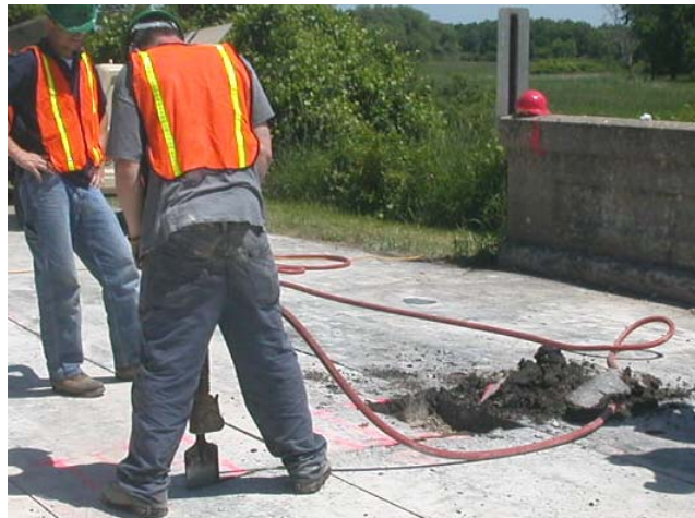
Figure 6.7. Removing the asphalt overlay
