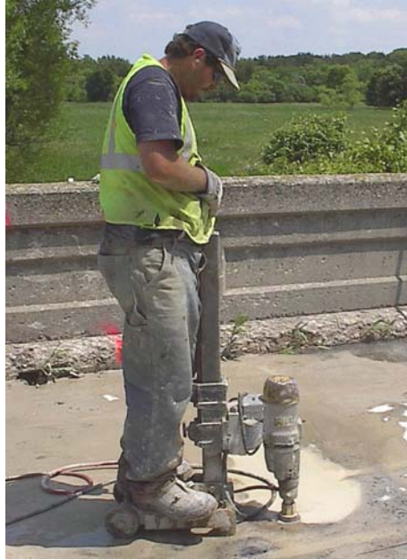
Figure 6.6. Contractor drilling through depth of bridge deck
