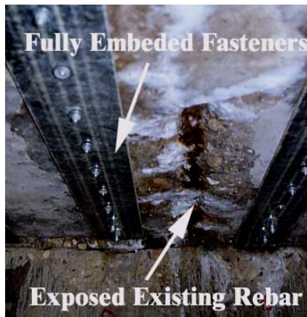
Figure 4.30. Existing damaged area in the bridge with the exposed steel reinforcement
