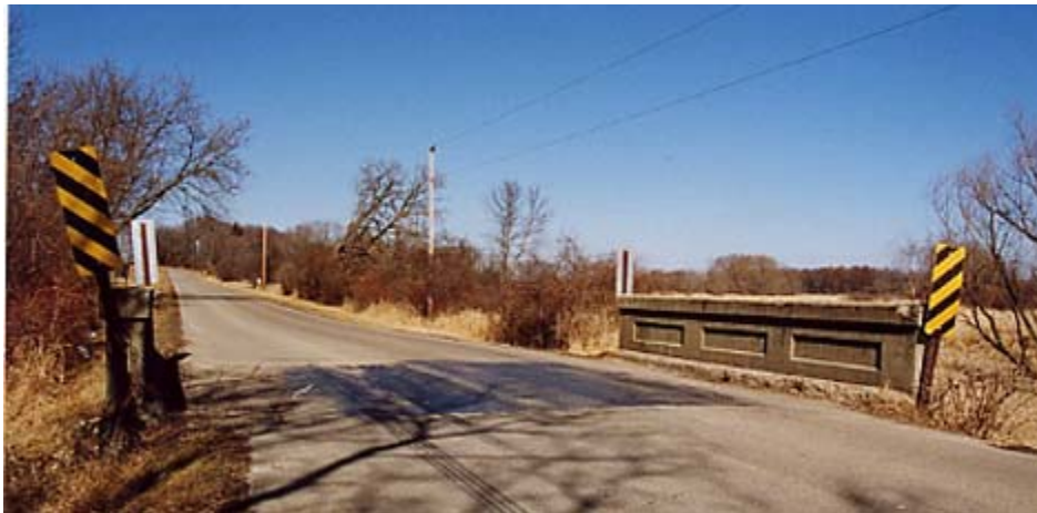
Figure 4.3. View of roadway of Bridge P-53-702
