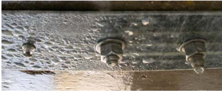
Figure 6.41. Stainless steel fasteners and anchors bolts
