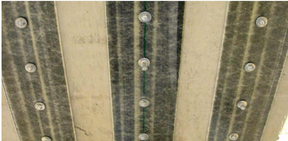
Figure 5.8. FRP 3 beam strengthened with three FRP strips
