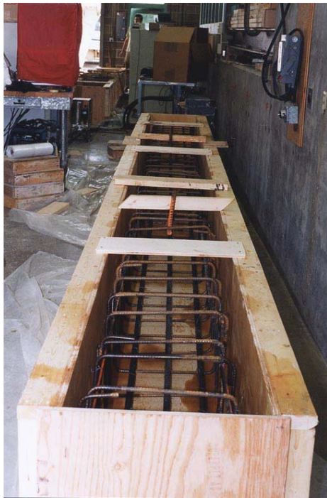
Figure 5.3. Formwork and reinforcement cages
