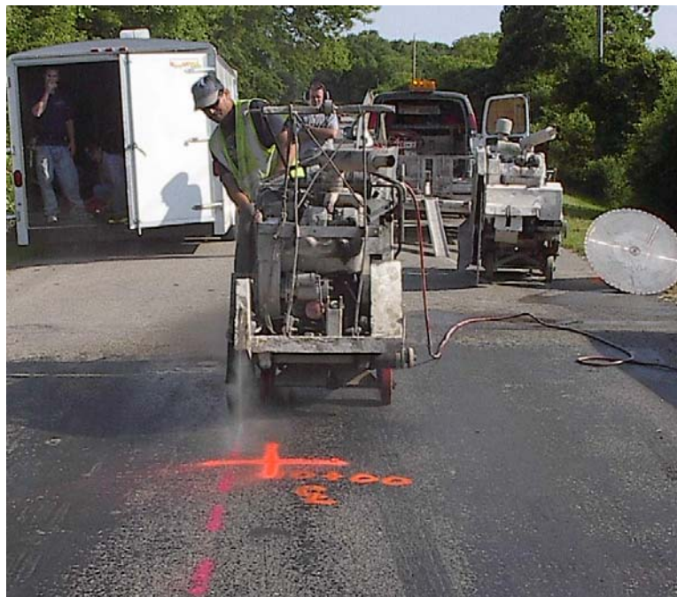
Figure 6.1. Contractor cutting the bridge deck (Cut #1)
