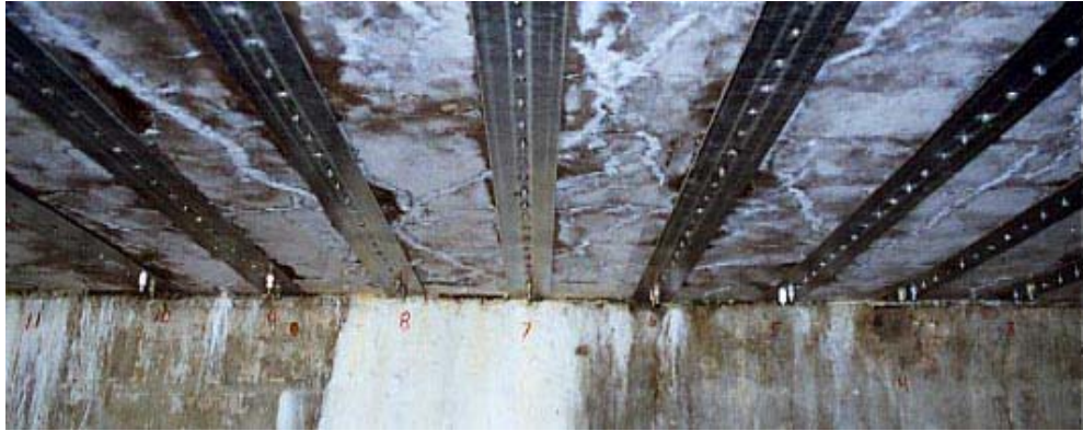
Figure 4.25. 12 in. Strip spacing between FRP strips
