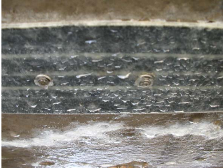
Figure 6.45. Edge of FRP strips covered with water
