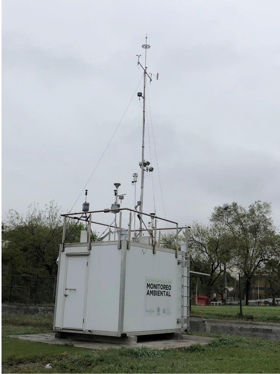
Figure 4 Monitoring station in San Nicolas de los Garza.
