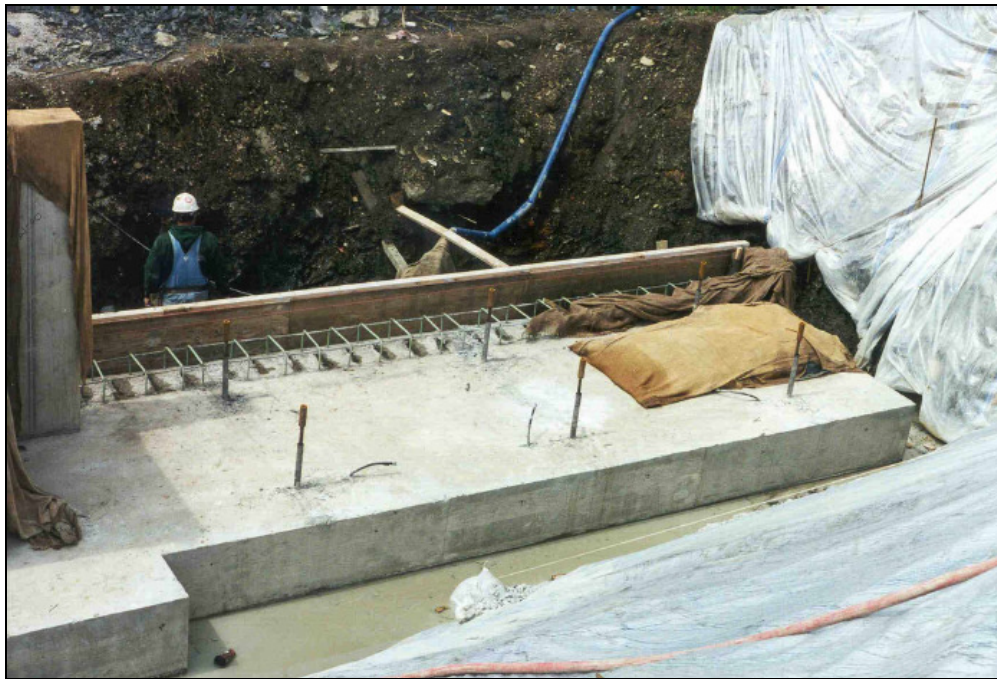
Figure 2-8 – Post-tensioning dowels in the footing 17
