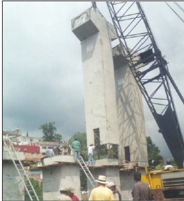
Figure 2-11 – Precast pier module with an hammerhead extension to form the pier cap later 20
