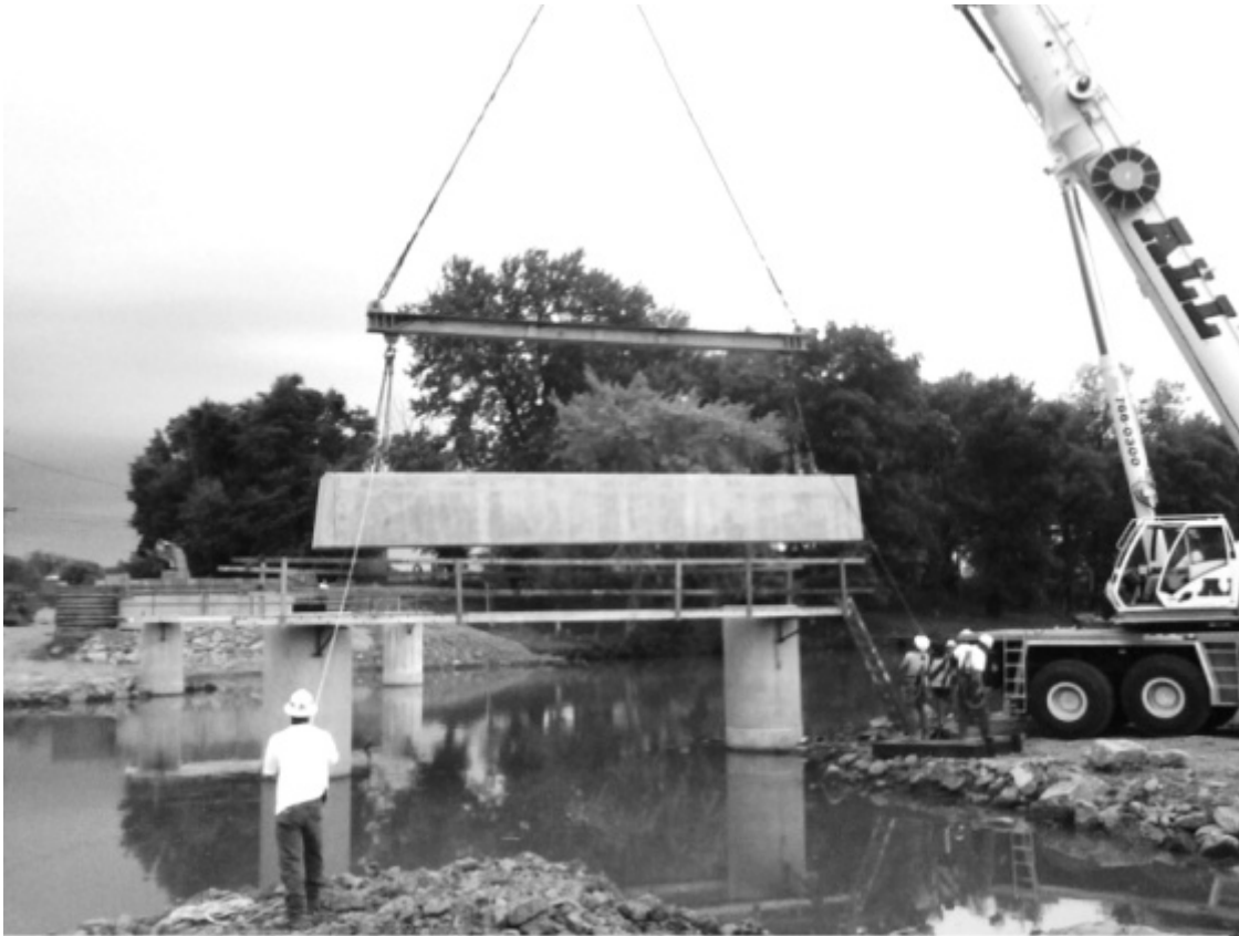
Figure 7-1 – Erection of Precast Pier Cap 40
