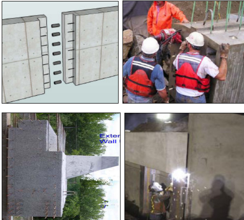
Figure 3-4 – Abutment module to module connection methods: Spliced Sleeves (top left), Post tensioning 37 (top right), Cast in place closure joints 12 (bottom left), Welding 11 (bottom right)
