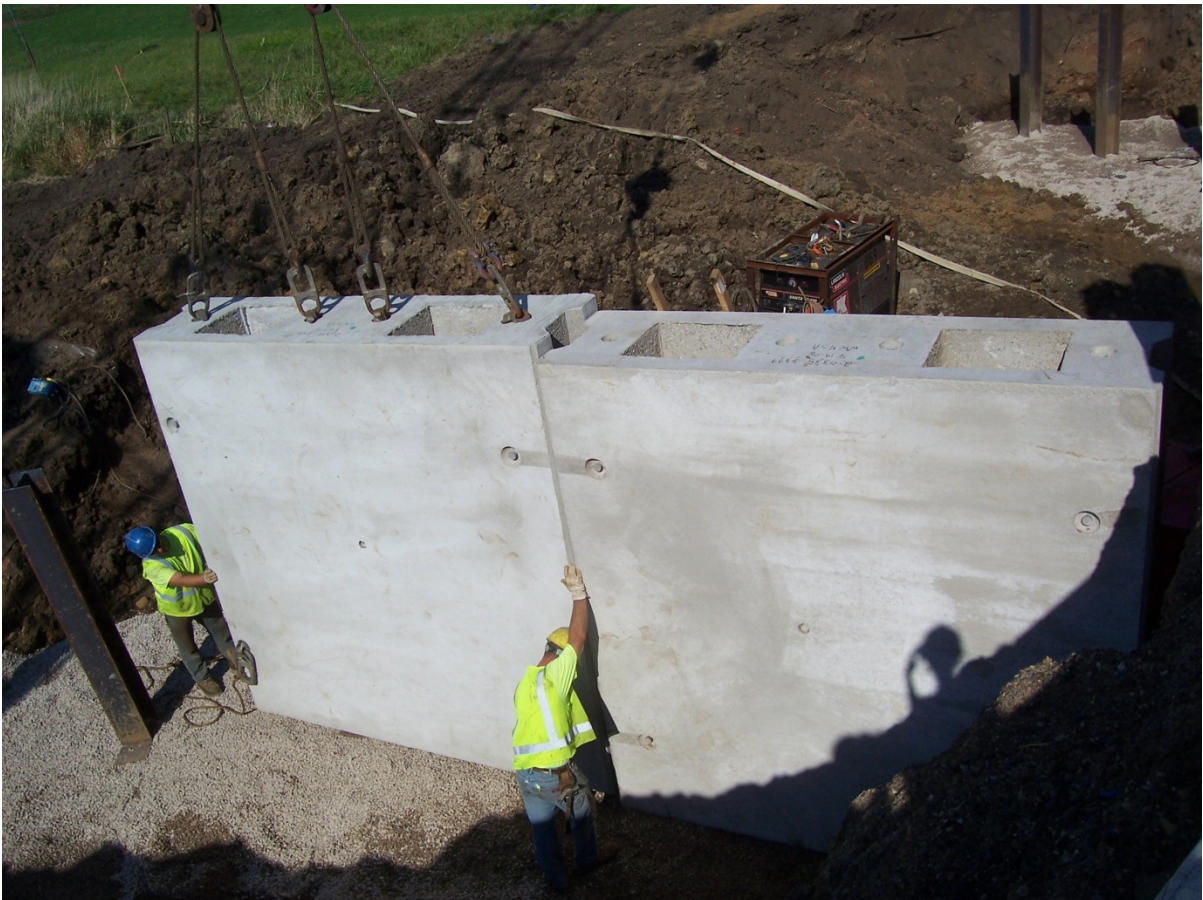
Figure 6-2 – Setting the second abutment module in place
