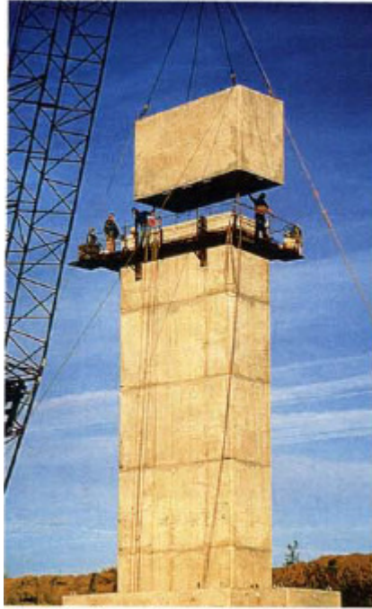
Figure 2-13 – Erection of precast box pier section 23
