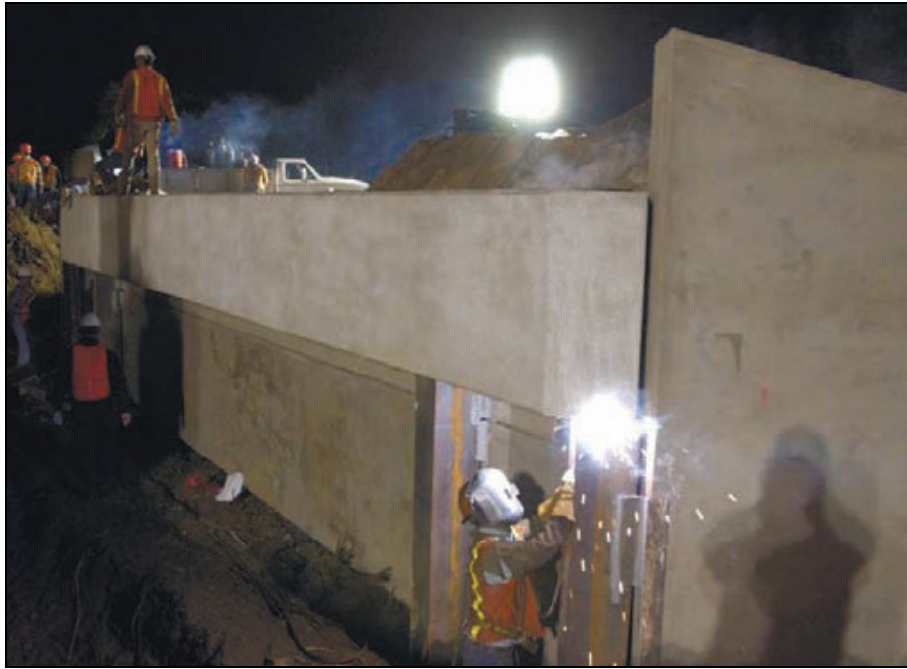
Figure 2-5 – Welding the precast modules together 11
