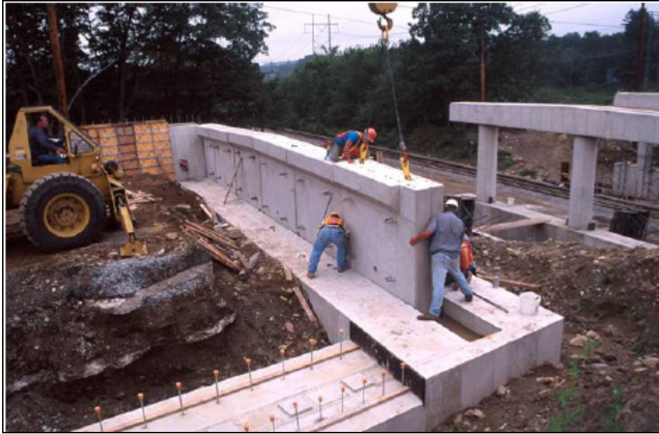
Figure 2-9 – Precast abutment pin connected to the footing 5
