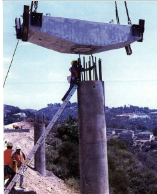
Figure 2-19 – Precast cross head with sleeves 31
