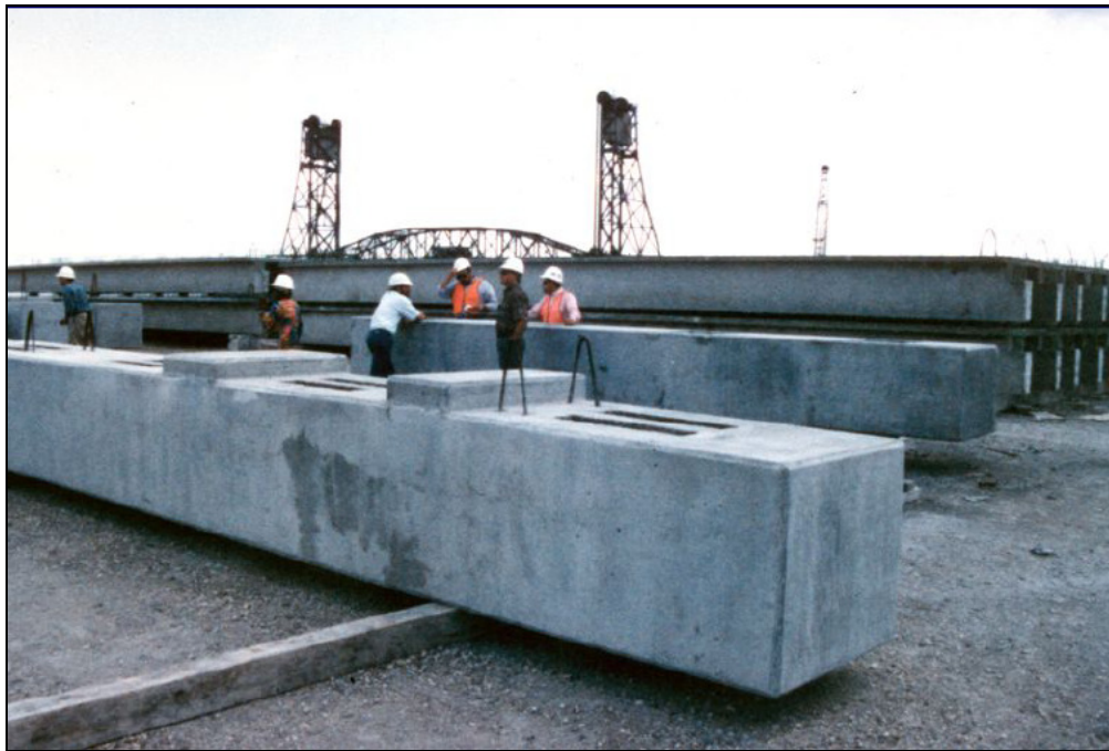
Figure 2-17 – Precast pile cap with pockets visible ready to accommodate the connectors 30
