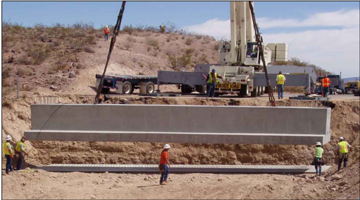
Figure 2-2 - Single piece abutment stem and partial footing 9
