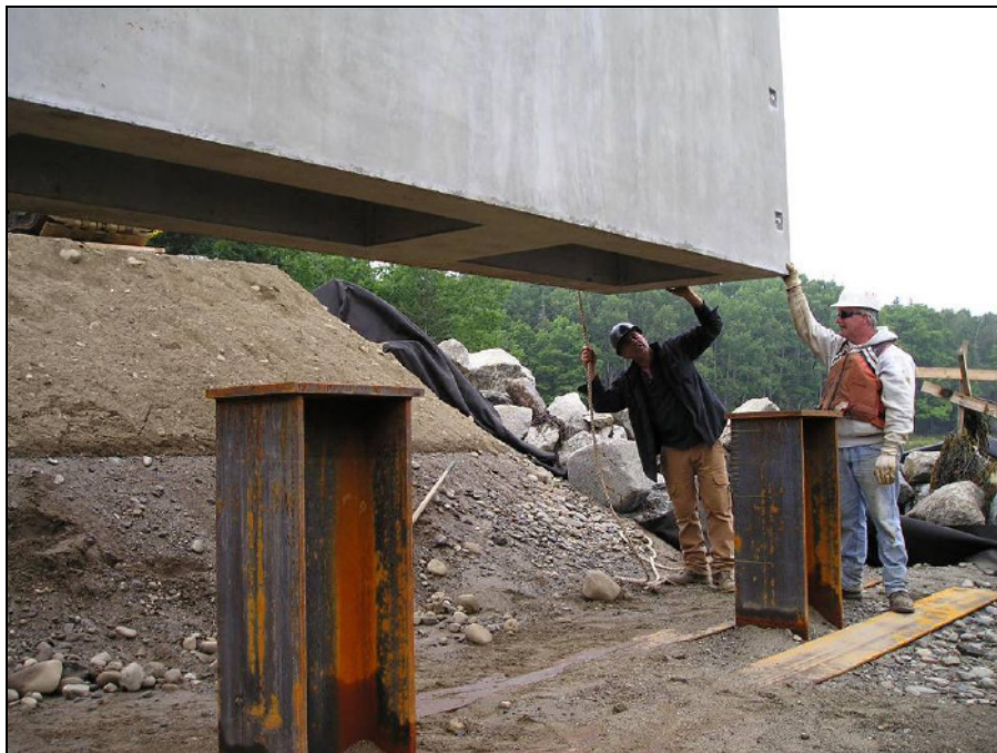
Figure 2-6 – Precast abutment with block-outs, being placed on steel H piles 15
