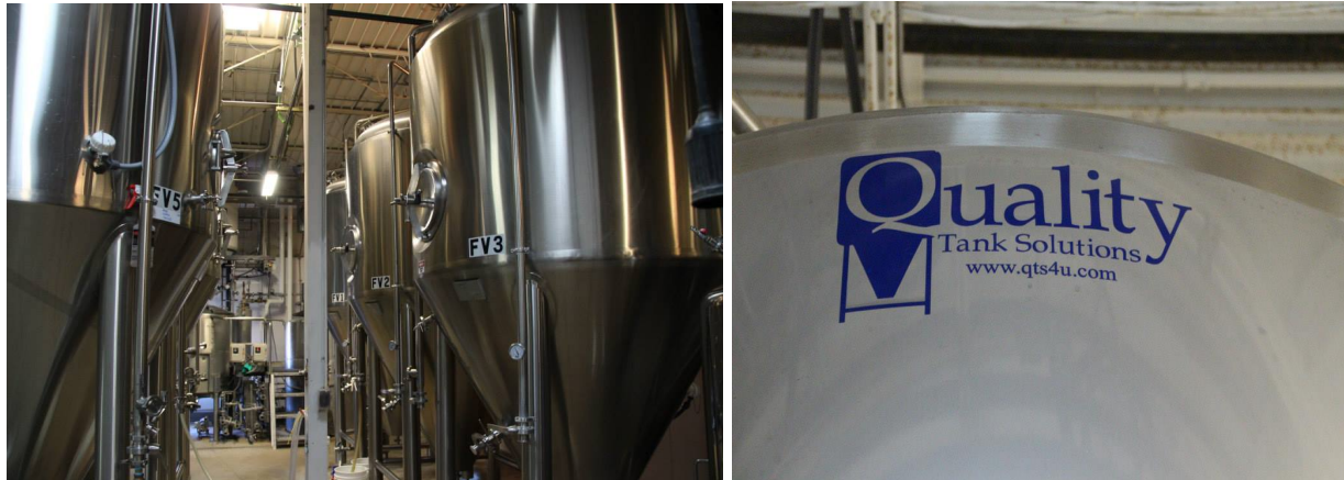
(Fermentation tanks from the brewing space at Karben4) (Photos: K. Zickert)
