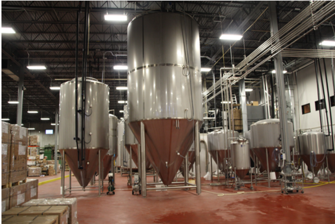
(Fermentation tanks in the new 45,000 square foot brewing space) (Photo: K. Zickert)
