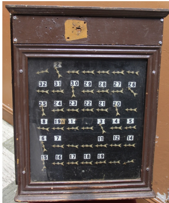
Figure 2.21. Original indicator board for the private booths, 2020. Photo by author.
