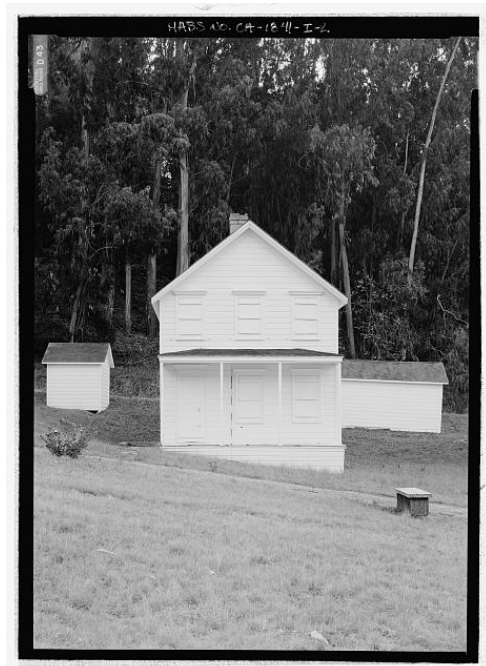
Figure 1.9. Elevation view of the northwest façade, same source as figure 1.8.
