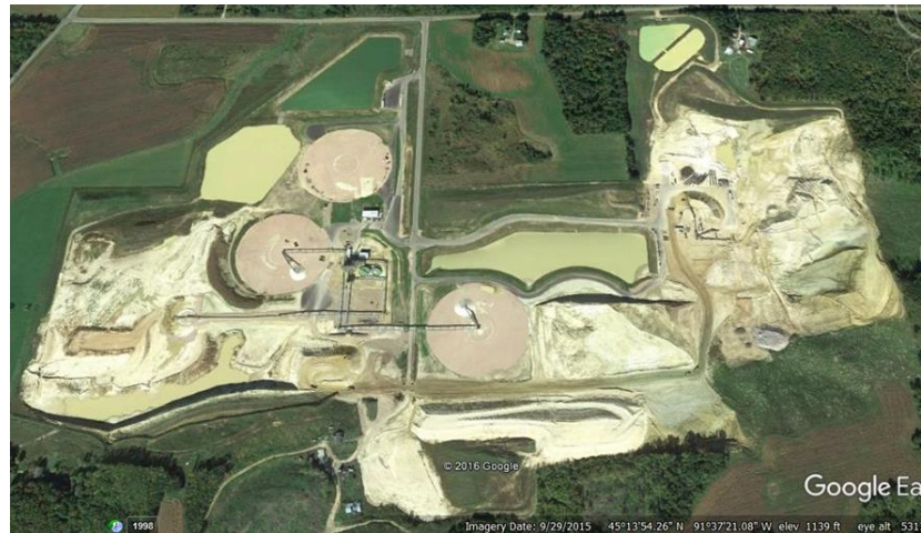
Figure 13 (9/29/2015) Close-up of the southern section of the New Auburn frac sand mine.
