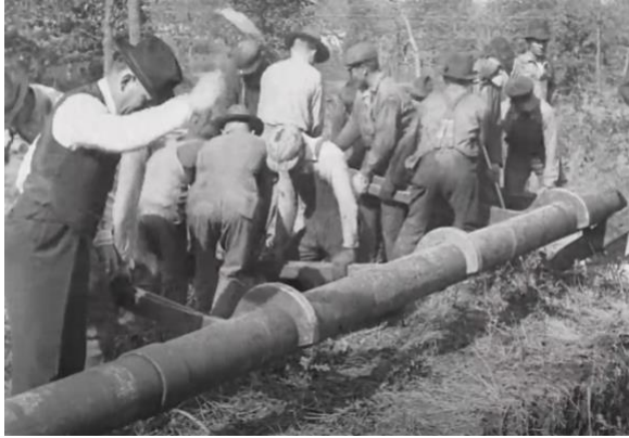
Figure 14 Workers laying pipe in S.o.P. (1923)
