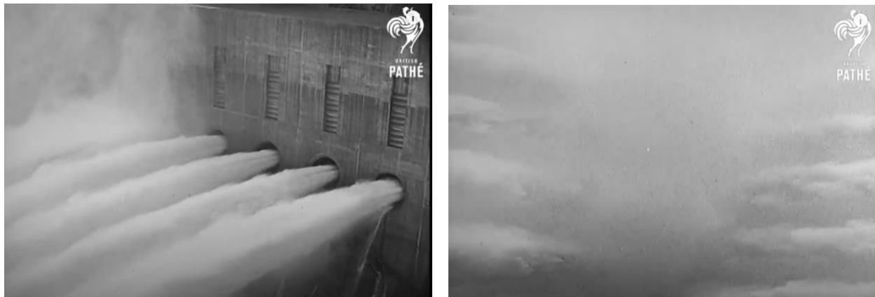
Figure 6 Boulder (Hoover) Dam diversion tunnels from different angles
