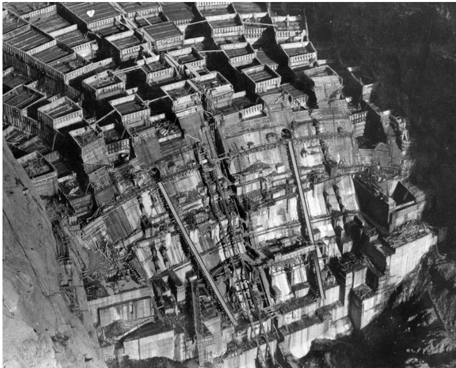
Figure 5 Boulder (Hoover) Dam under construction in February 1934.
