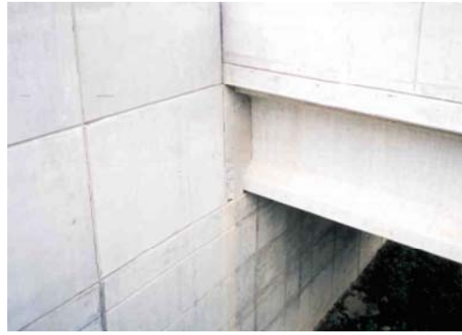
Figure 2.9 “Fixed End” Restraint (Saadeghvaziri and Hadidi 2002).
