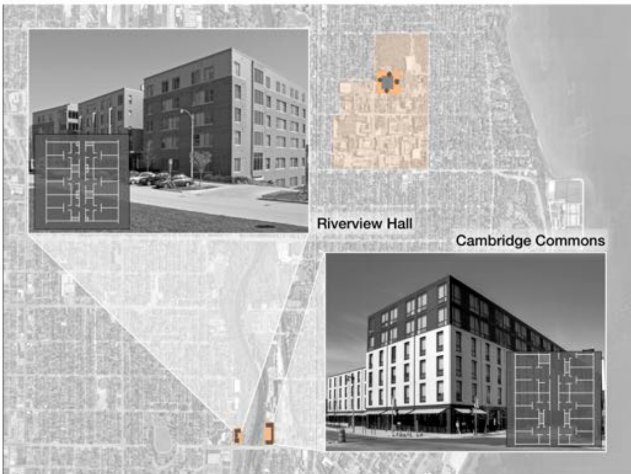
Figure 15. Riverview Residence Hall and Cambridge Commons.
