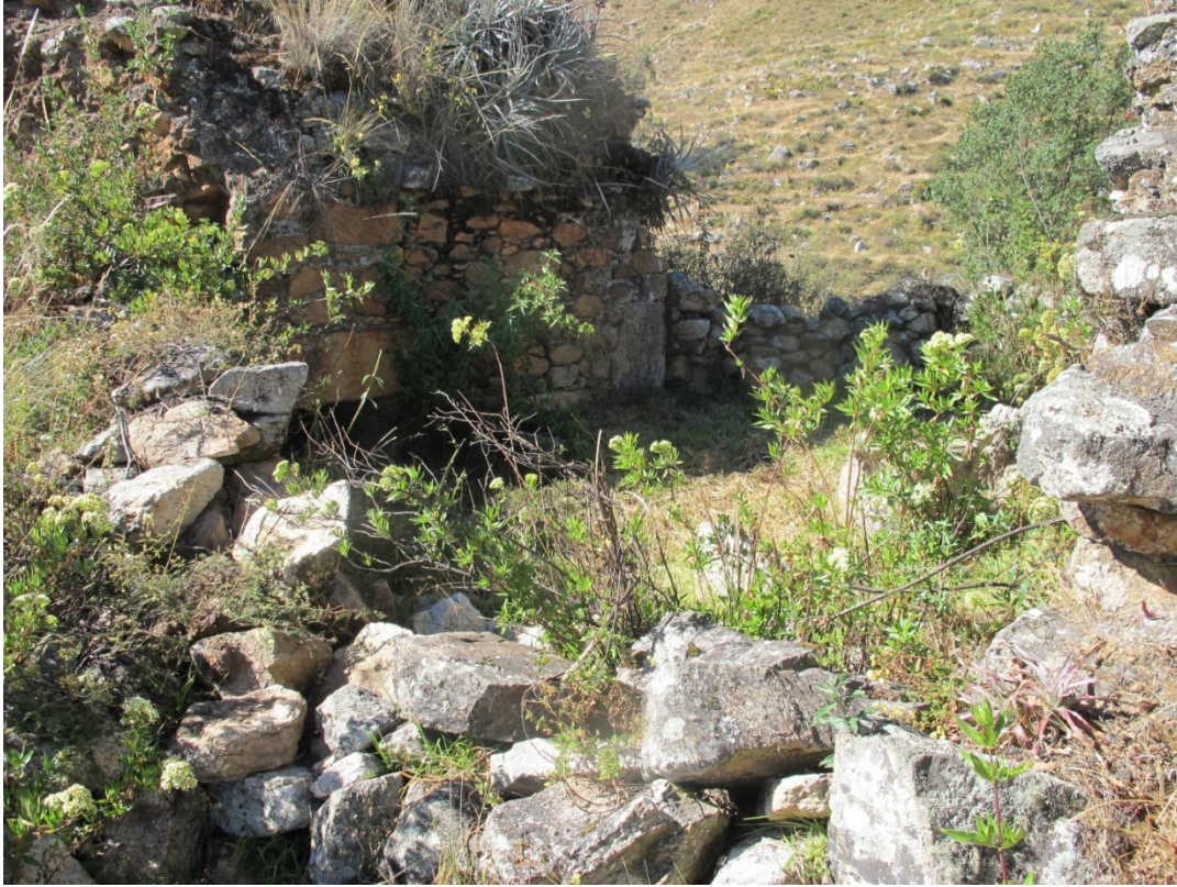
Figure 12. Low wall creating enclosed space around entrance of Chullpa 40.
