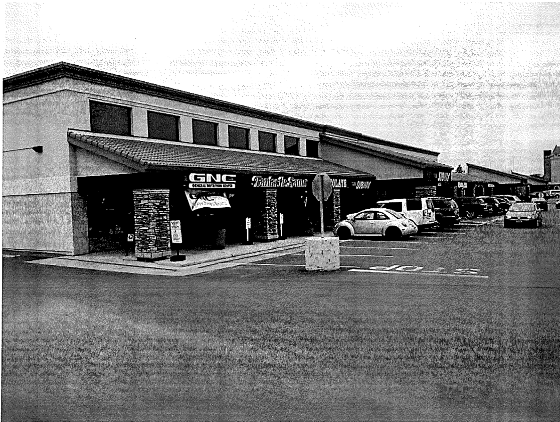
Image 2. Northeastern corner of Miracle Mile, March 25, 2017. Photograph by Lauren Anderson. This is the eastern section of the shopping center, otherwise known as the Excel Building.
