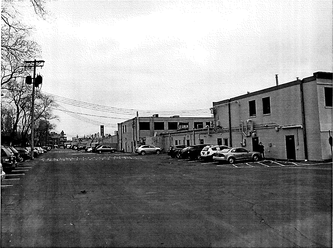
Image 9. Rear elevation of Miracle Mile, March 25, 2017. Photograph by Lauren Anderson.
