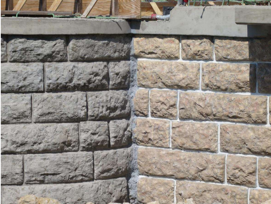
Figure 3-1: Prepared and coated form lined concrete surfaces.
