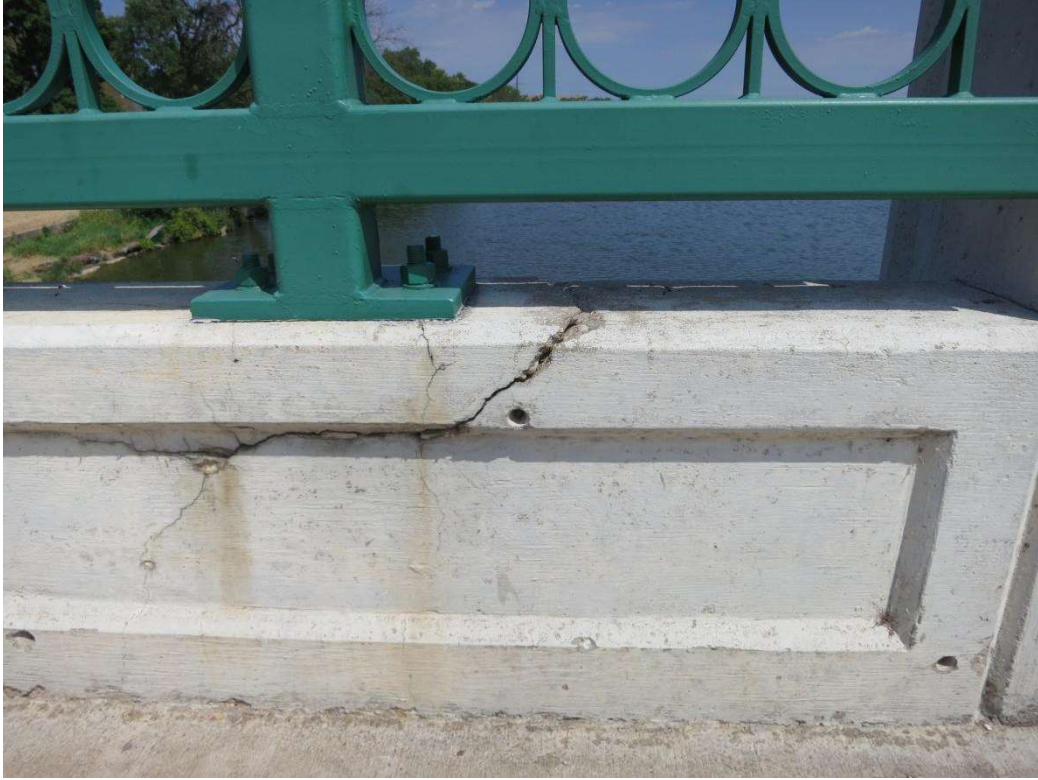
Figure 3-6: Voids left in concrete surface to accommodate form ties.
