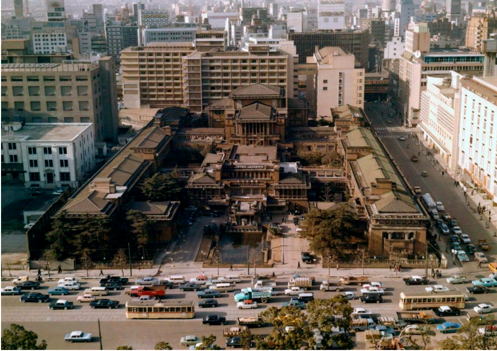
Figure 3.54. Imperial Hotel, Tokyo, shortly before demolition.
