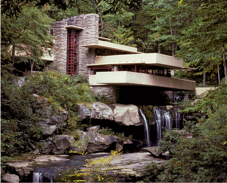
Figure 2.1 Frank Lloyd Wright, Fallingwater. 1937.
