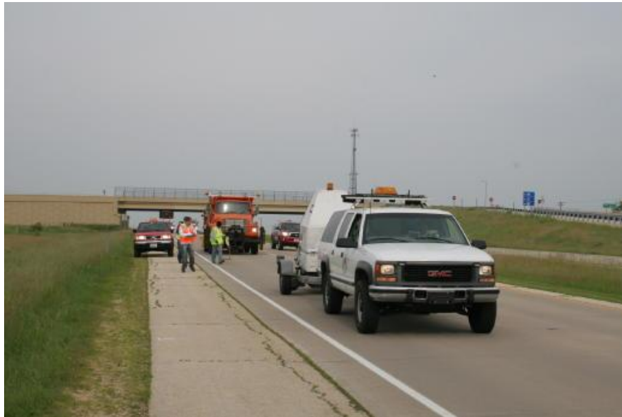
Figure 4.3 FWD Testing on USH 18/151 at Barneveld Interchange
