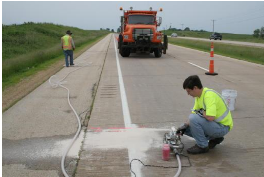
Figure 4.7 Water Inflow at Corehole and Recording Rate and Total Volume (USH 18/151)
