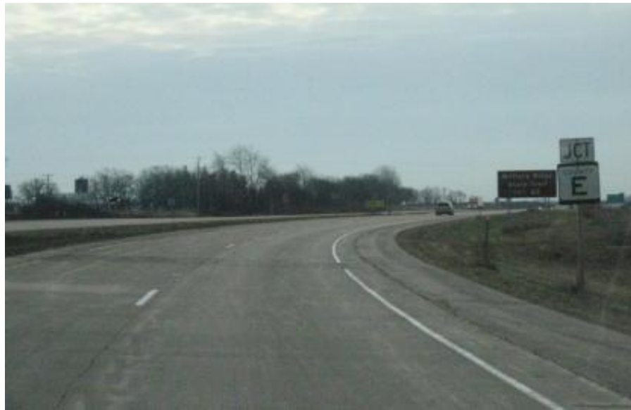
Figure 7.5 Patching on Doweled Dense-Graded Test Section #14 on USH 18/151
