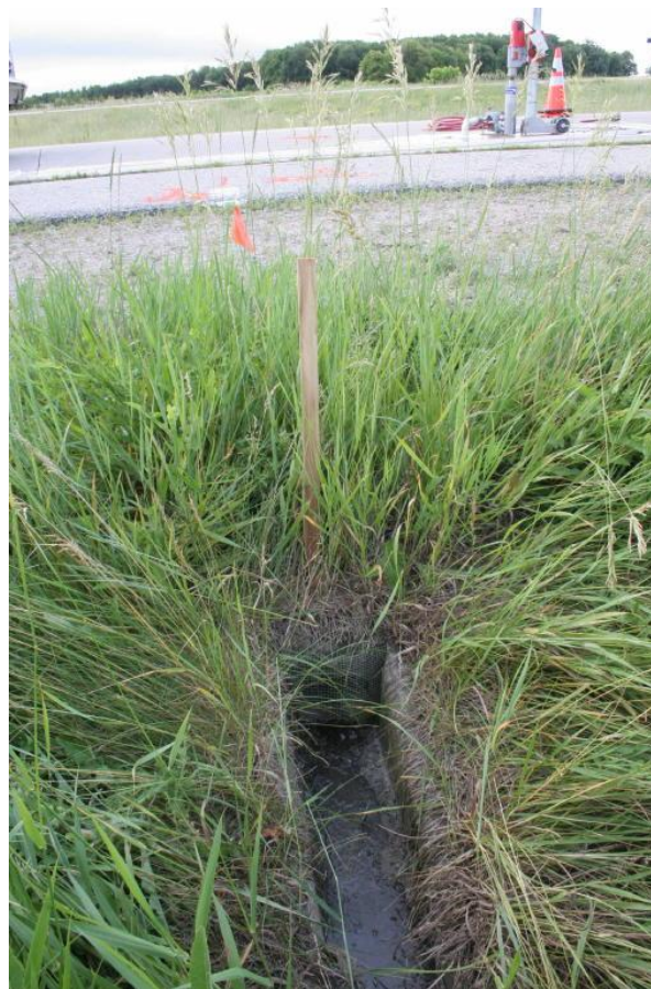
Figure 4.11 Water flowing out Edgedrain Pipe and Apron Endwall (STH 29)
