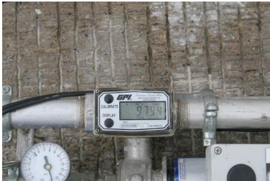
Figure 4.10 Flow Meter measuring 97.94 Gallons of Water into Corehole (STH 29)
