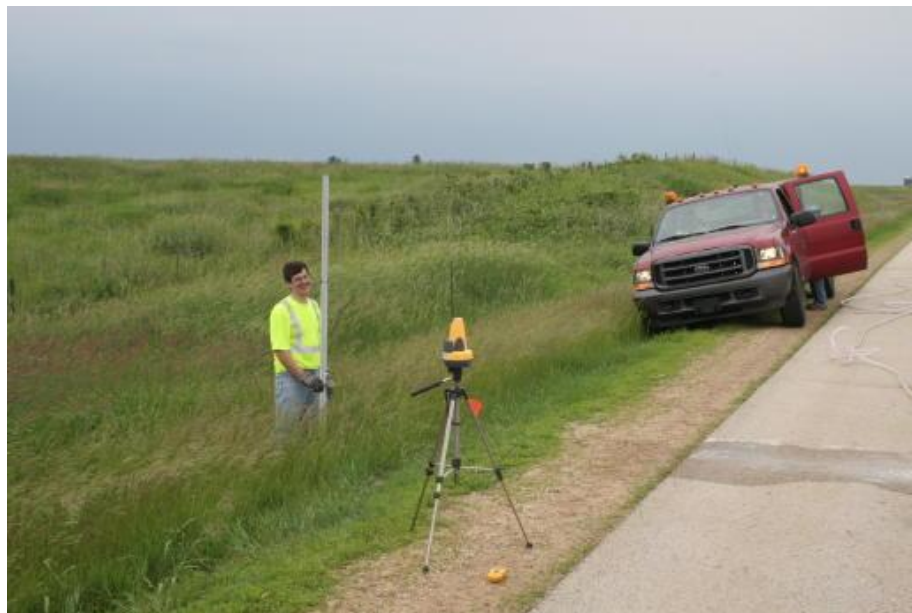
Figure 4.9 Recording Elevation at Outflow Drainpipe (USH 18/151)
