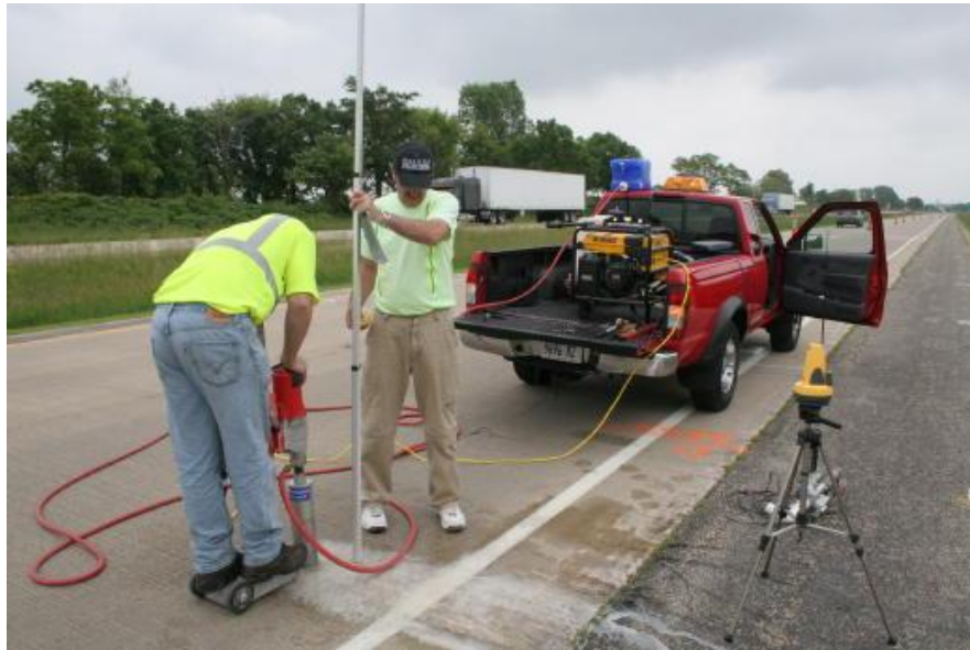
Figure 4.6 Drilling Corehole and Recording Elevations (USH 18/151)
