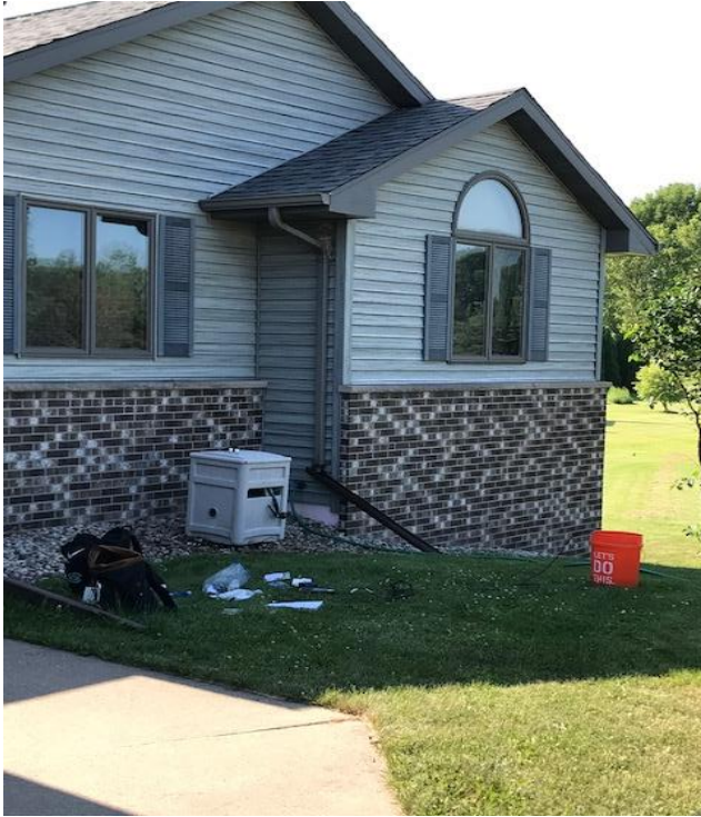
Figure 24. 1-hour pump test at location L9.
