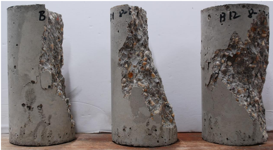
Figure I.5. Failure pattern of Cylinders 10, 11, 12 at 21 days
