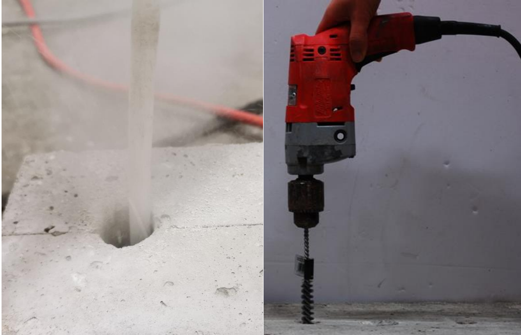
Figure V.5. Hole cleaning with a hand pump air blower and a wire brush
