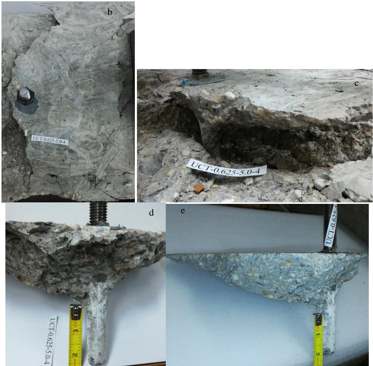
a) load-displacement behavior; b) cracked surface; c) concrete breakout cone in block; d) e) concrete breakout cone.
