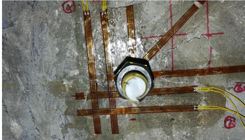
Figure 6.13. Strain gages installed on concrete surface.
