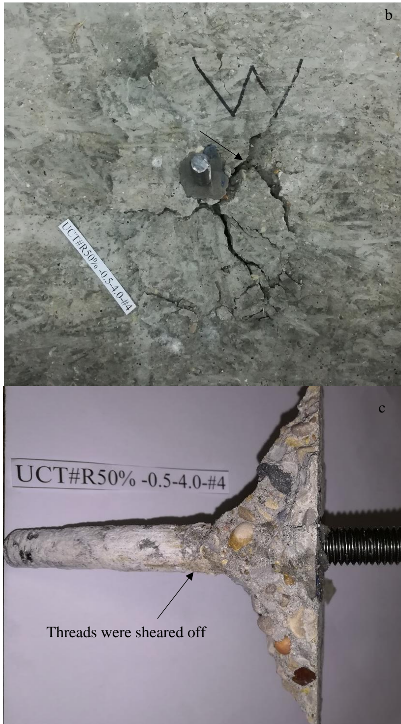
a) load-displacement behavior; b) cracked surface; c) partial cone bond failure Figure VI.32. Observed behavior of Specimen UCT#R50%-0.5-4.0-#4
