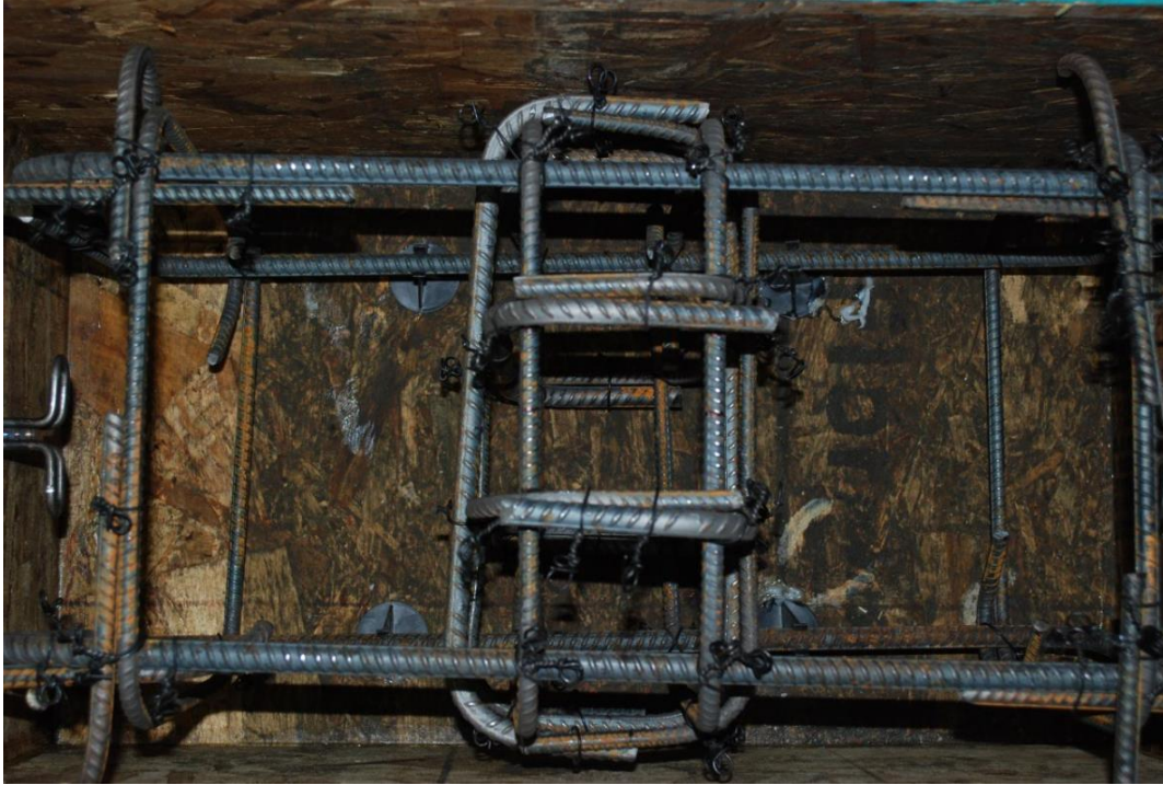
Figure 4.5. Pictures of anchor reinforcement for unconfined pullout tests
