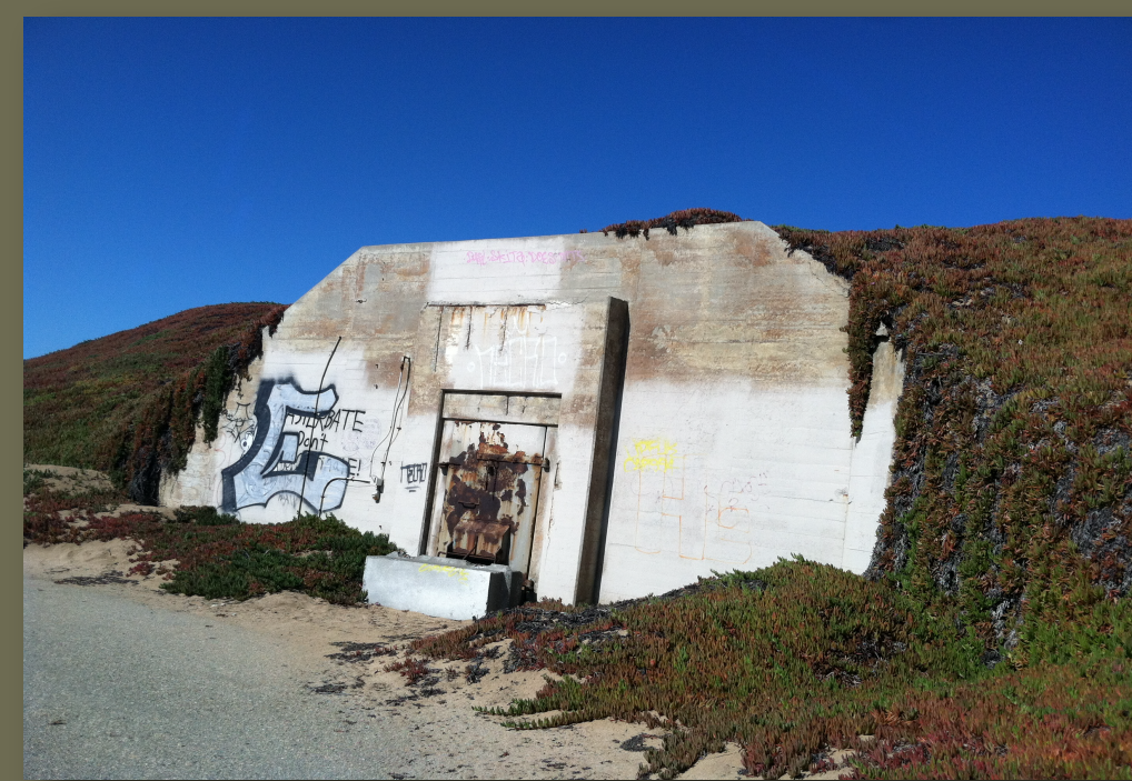
Figure 2: Embedded ammunition bunker
