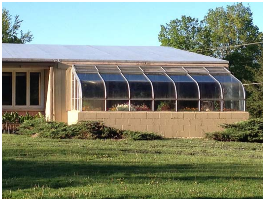
Figure 6 – Greenhouse connected to the classroom
