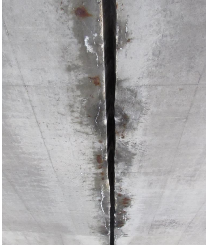
Figure 4.13 - Efflorescence and corrosion due to retained moisture at waterstop joint between adjacent bridges. (B-30-025/026)
