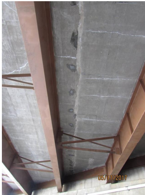
Figure 4.8- Transverse cracks extending to abutment in Stage 2 deck (right side). Transverse cracks in Stage 1 deck (left side) only near midspan region. (B-70-176)
