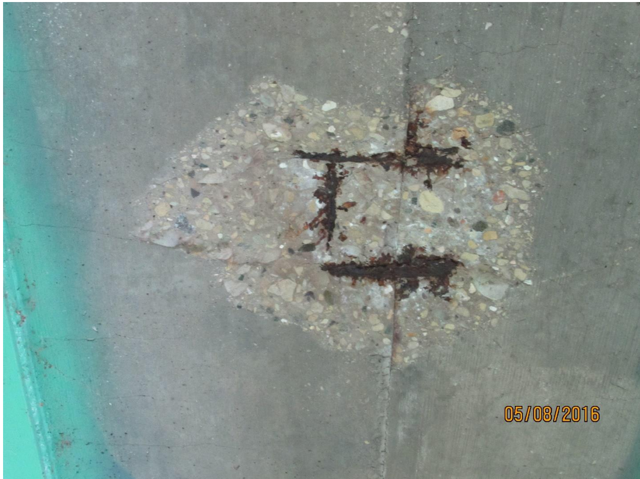
Figure 4.7- Spalled concrete and corroded reinforcement. Transverse cracking at approx. same spacing as transverse reinforcement (B-13-593)
