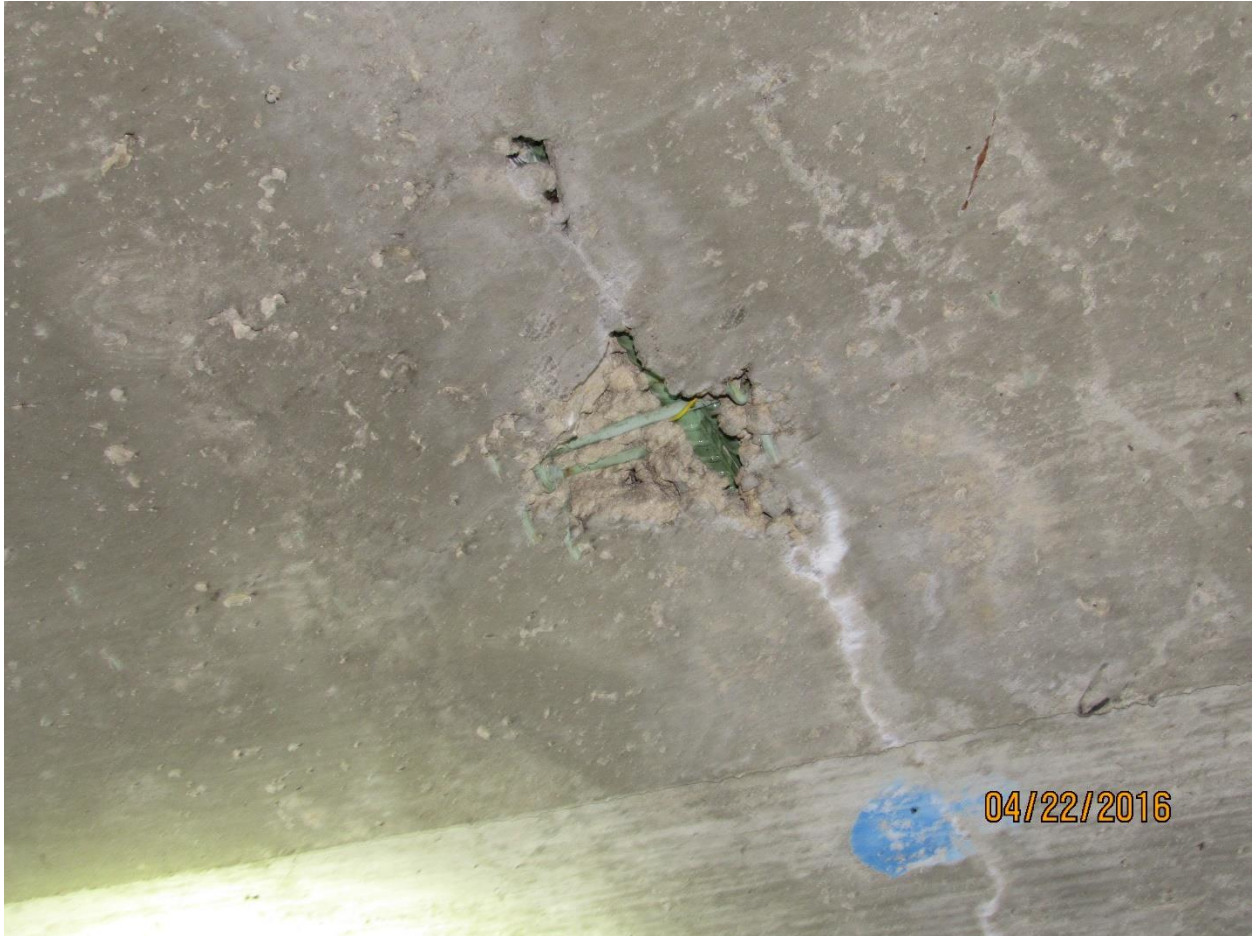
Figure 4.2- Inadequate concrete consolidation exposing reinforcement in the longitudinal joint region. (B-40-216 – Dowel bar splicer; detail B per Figure 4.1)
