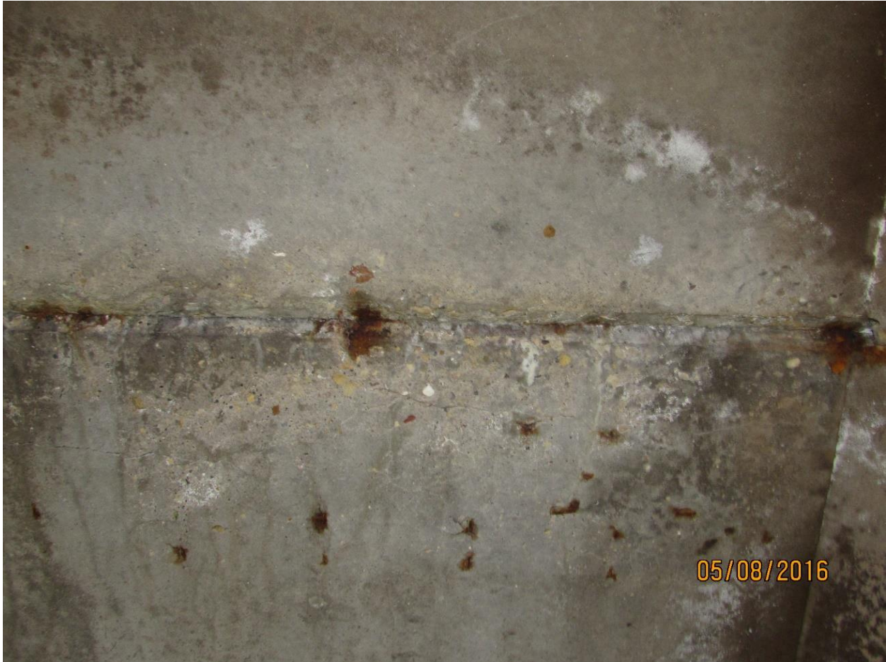
Figure 4.6 - Typical spots of corrosion on the underside of the longitudinal construction joint (B-56-022)
