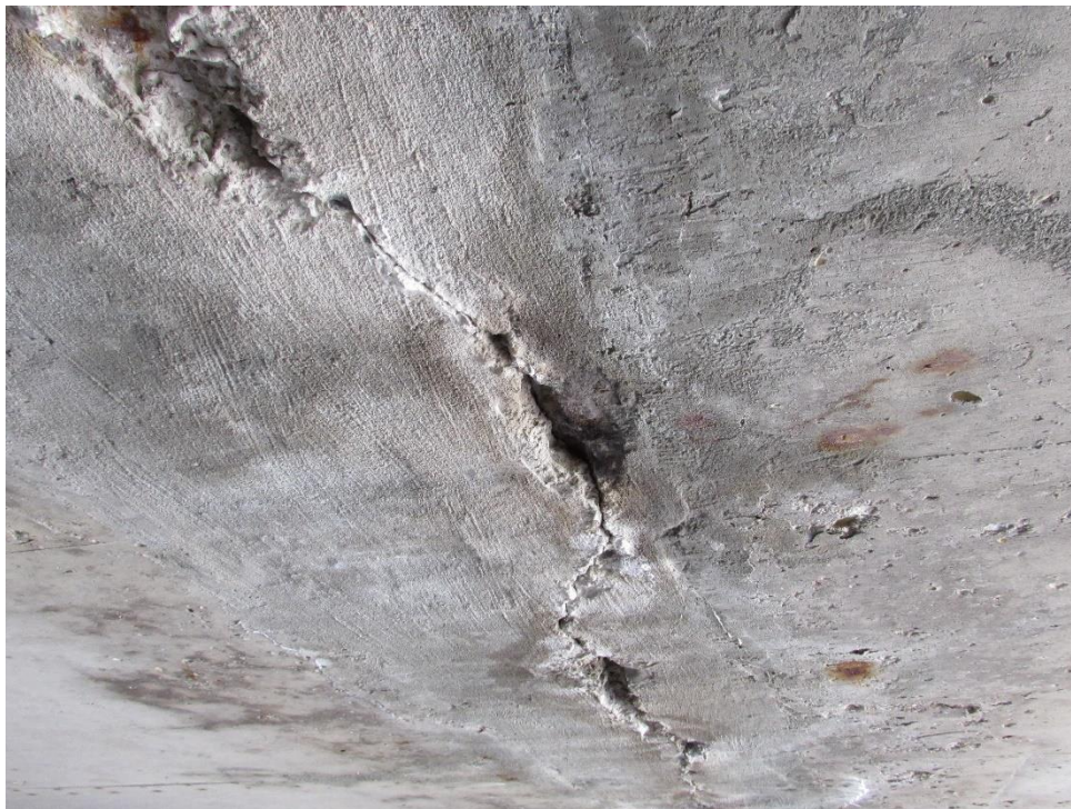
Figure 4.14 - Large longitudinal crack opening approximately 1/4" during the passage of large trucks. (B-30-015)
