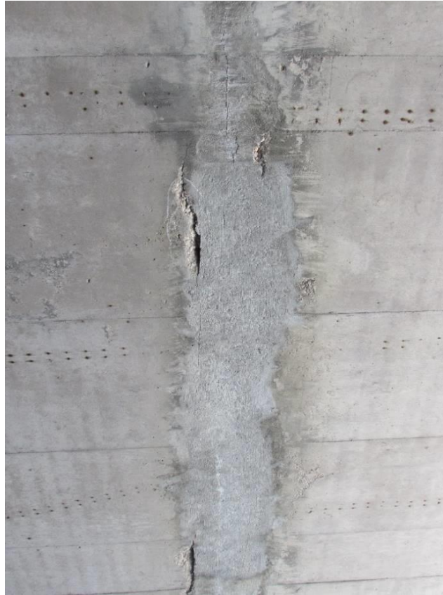
Figure 4.9- Patching of previously spalled concrete at longitudinal construction joint in haunched slab bridge. (B-30-026)
