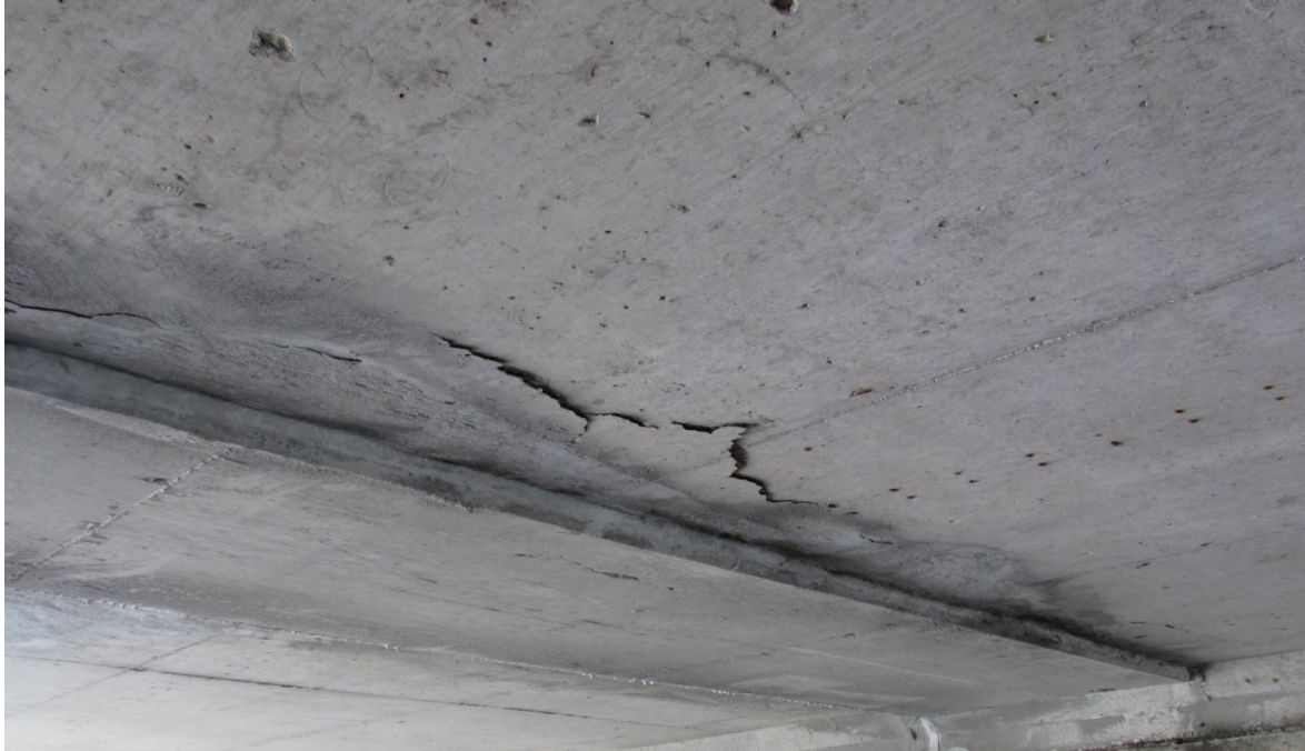
Figure 4.12 - Delaminated area adjacent to longitudinal construction joint in widened portion of deck. (B-30-014)
