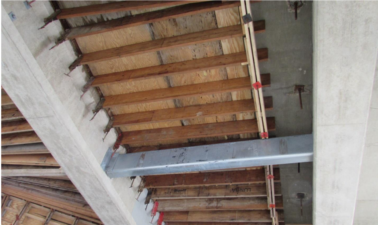
Figure 7.9 - Formwork system as seen in staged construction of bridge B-64-123. Wood beams are supported by top flange of left girder and rods are drilled through Stage 1 hardened deck on right side.
