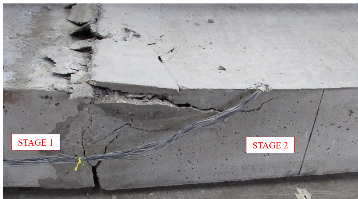
Figure 7.31 - Specimen 2 compression block failure at construction joint.
