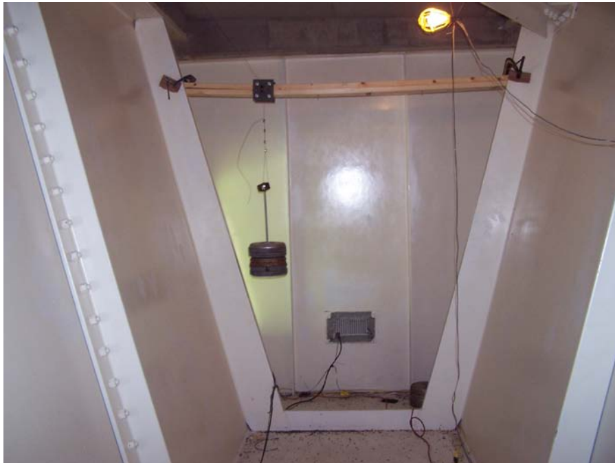
Figure 3.9: South End of Bridge Girder
