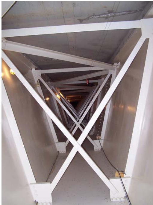
Figure 3.2: View Inside Bridge Girder
