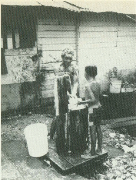
This pump in the Curundu area of Panama City served for drinking water, cooking and laundry needs.
