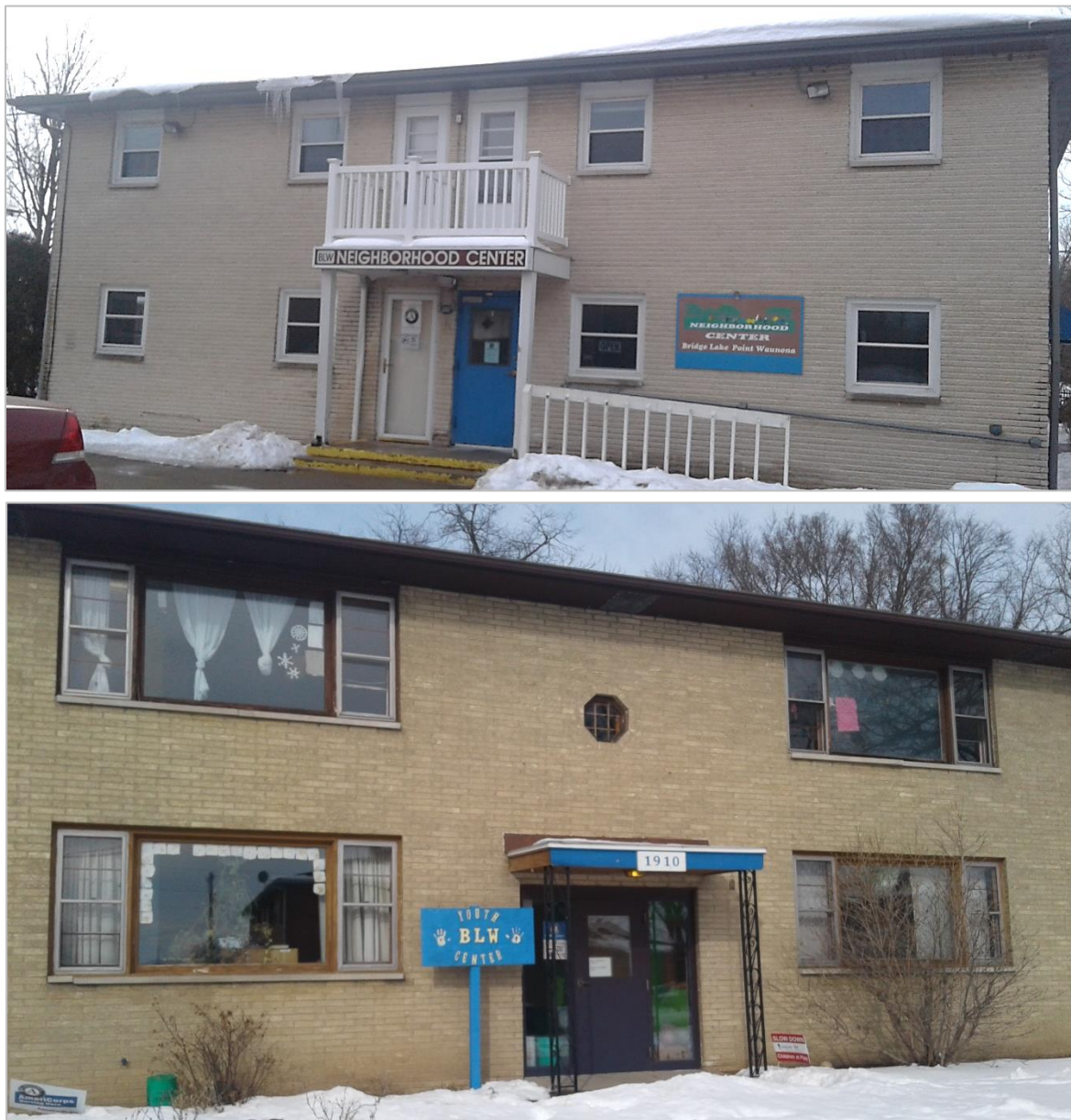
Figure 3.3 The BLW Center's main building (top) consists of the converted first floor space that sits below occupied apartments. The apartment residents and the BLW Center share a 10-car parking lot and a small playground. Across the street sits the BLW Youth Center (bottom), which occupies the full 2-story apartment building with basement, 3-car parking lot in the rear, and small play yard.
