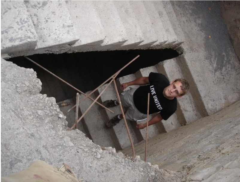
Figure 9: Learner Observes Unfinished Construction. Source: Learner's photo.
