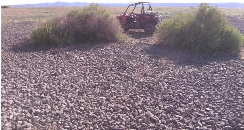
Figure 37 – Clockwise from top left: 1. Unvegetated riprap erosion cover. 2. Grasses growing in the riprap cover layer. 3. Ant mound protruding from the riprap cover (Test Pit 6). 4. Salt bush growing from the riprap layer (ATV for scale).
