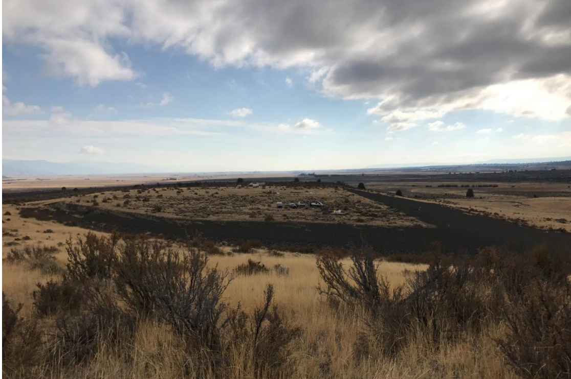
Figure 119 – View of the Lakeview, OR disposal cell looking south.
