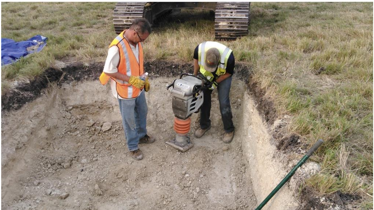
Figure 12 – Replacement and compaction of Rn barrier material.
