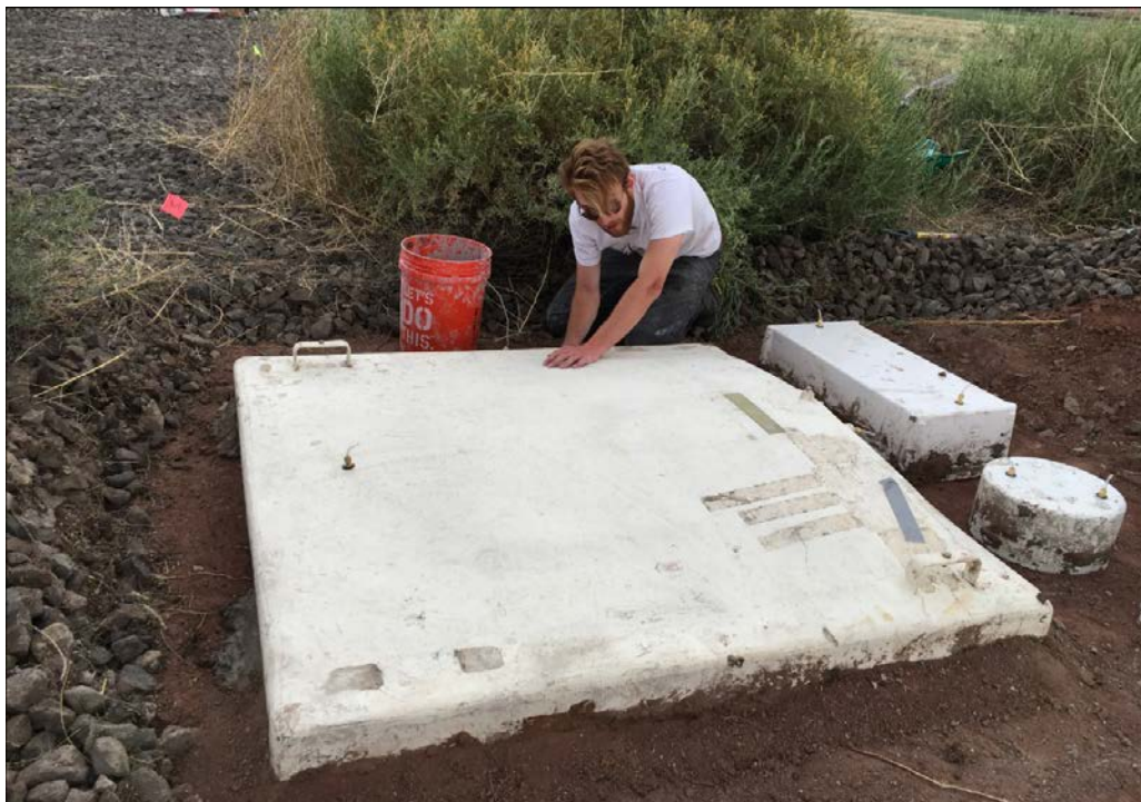
Figure 4.8 – Installation of flux chambers on the Rn barrier surface.
