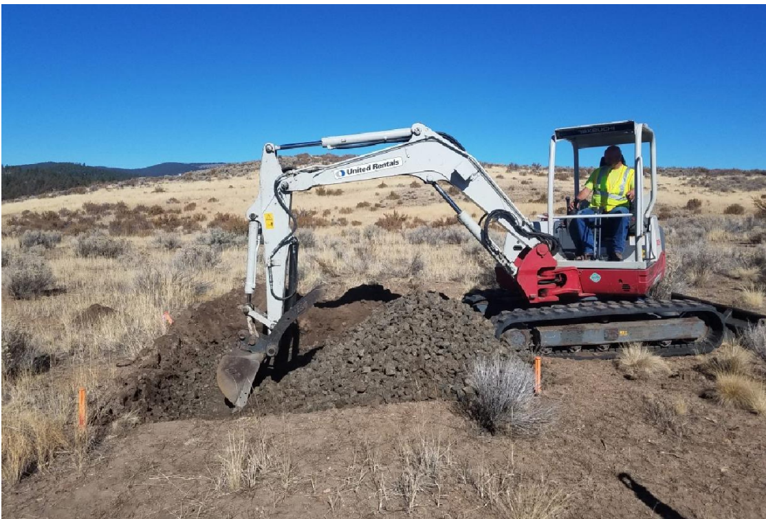
Figure 131 – Removal of the rip-rap layer.
