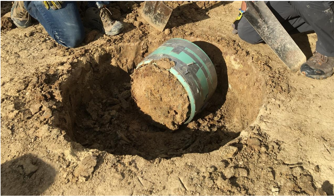
Figure D101 – 350 mm diameter sample after removal.
