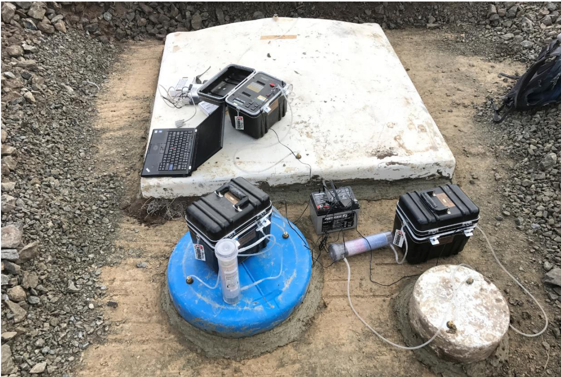
Figure 136 – Flux chambers installed on the Rn Barrier surface.
