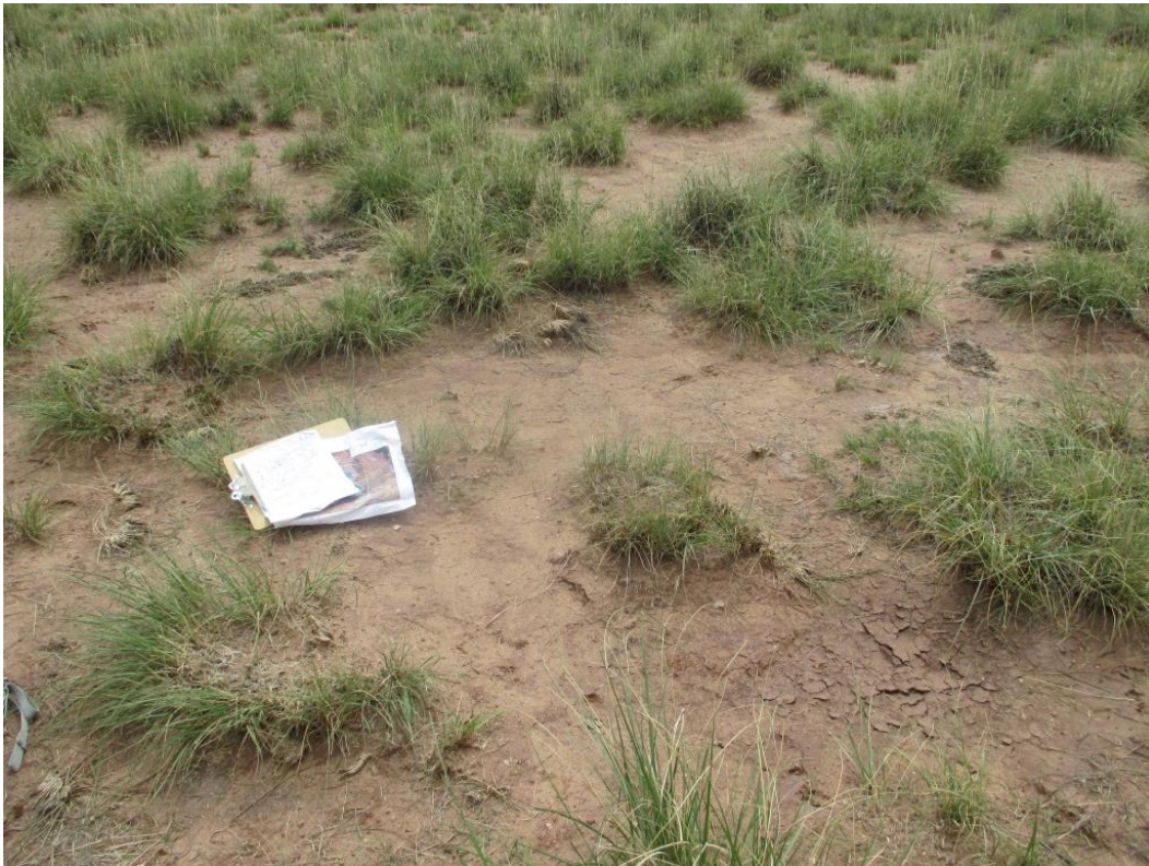
Figure 38 - Vegetated topsoil cover at the acid tailings pile disposal cell.
