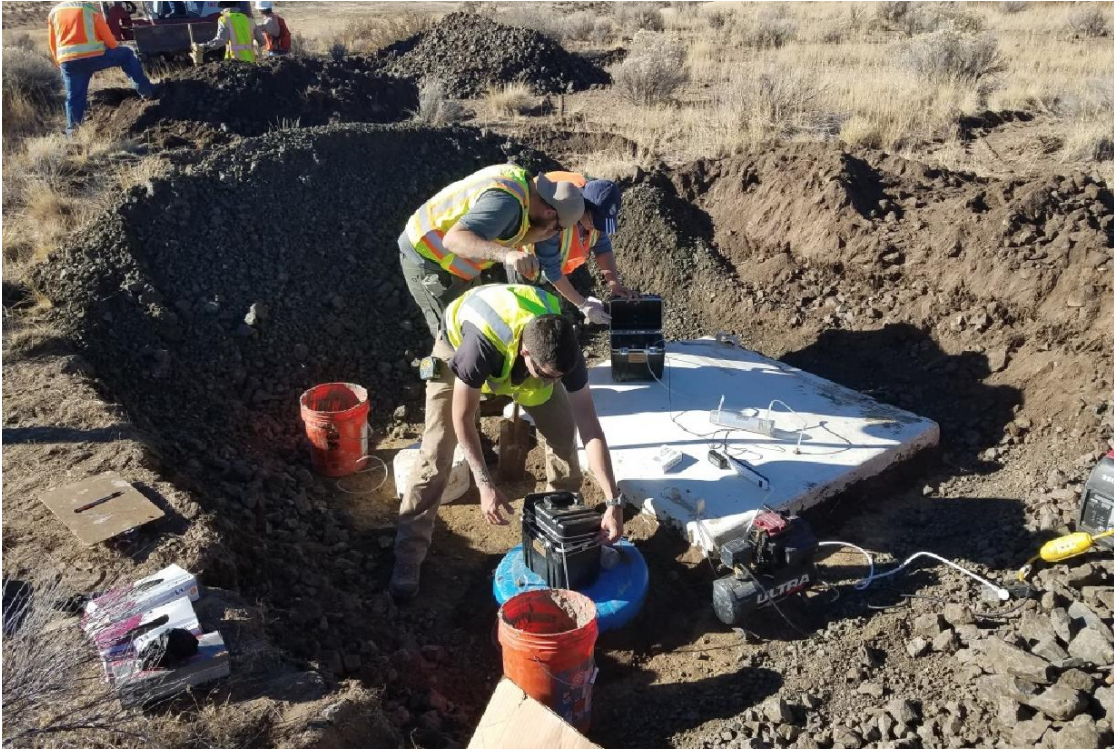
Figure 135 – Installation of flux chambers on the surface of the Rn barrier.
