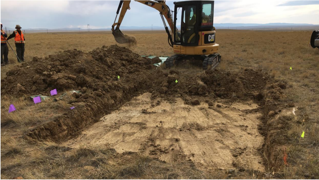
Figure B91 – Removal and stockpiling of the topsoil layer to expose the sandy overburden layer.
