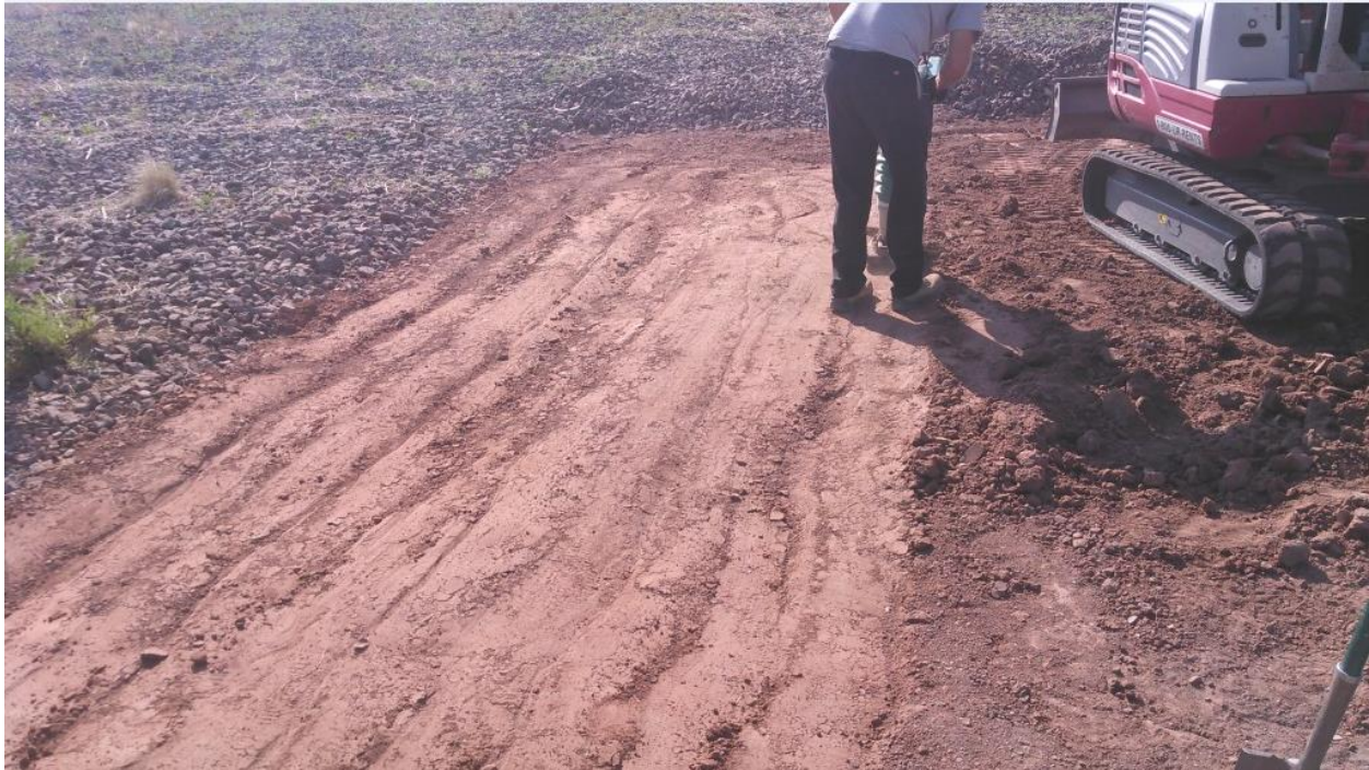
Figure 47 – Repair and compaction of the Rn barrier soil.
