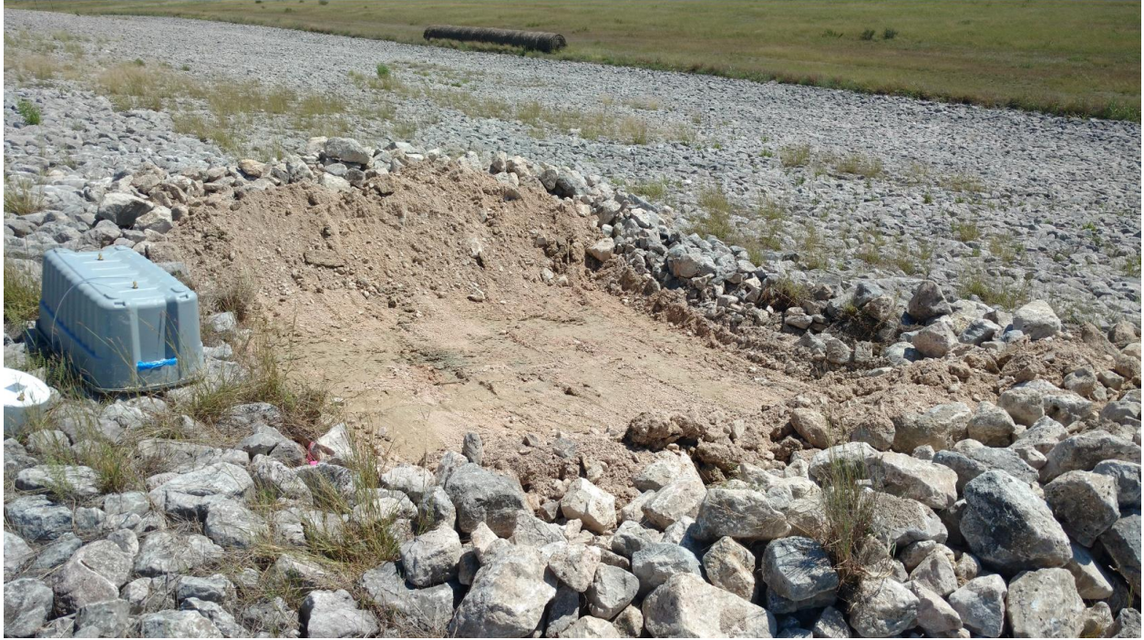
Figure 11 – Test pit with rip-rap layer removed to expose Rn barrier.
