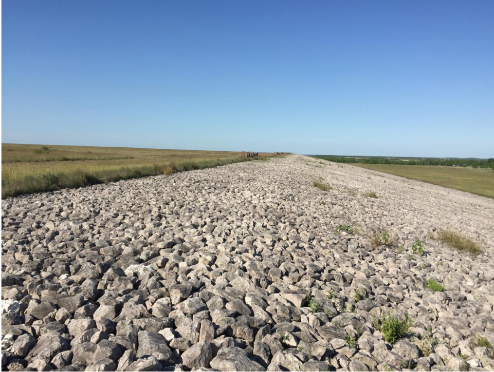
Figure 5 – Riprap on 5:1 slope.
