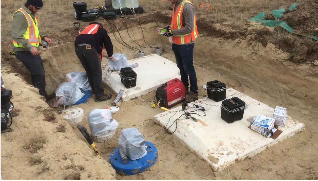
Figure C94 – Installation of flux chambers on the Rn Barrier surface.
