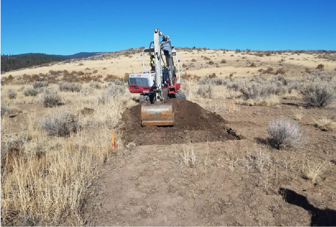
Figure 130 – Removal and stockpiling of the topsoil layer.
