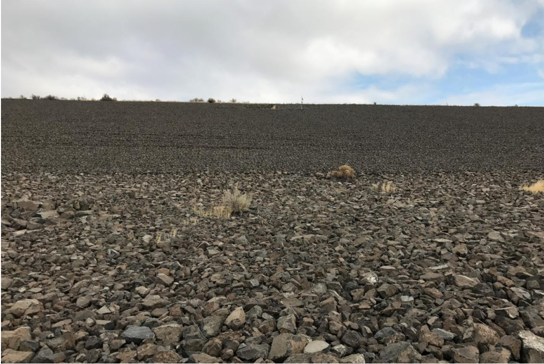
Figure 125 - Riprap covered slope of the disposal cell looking East.
