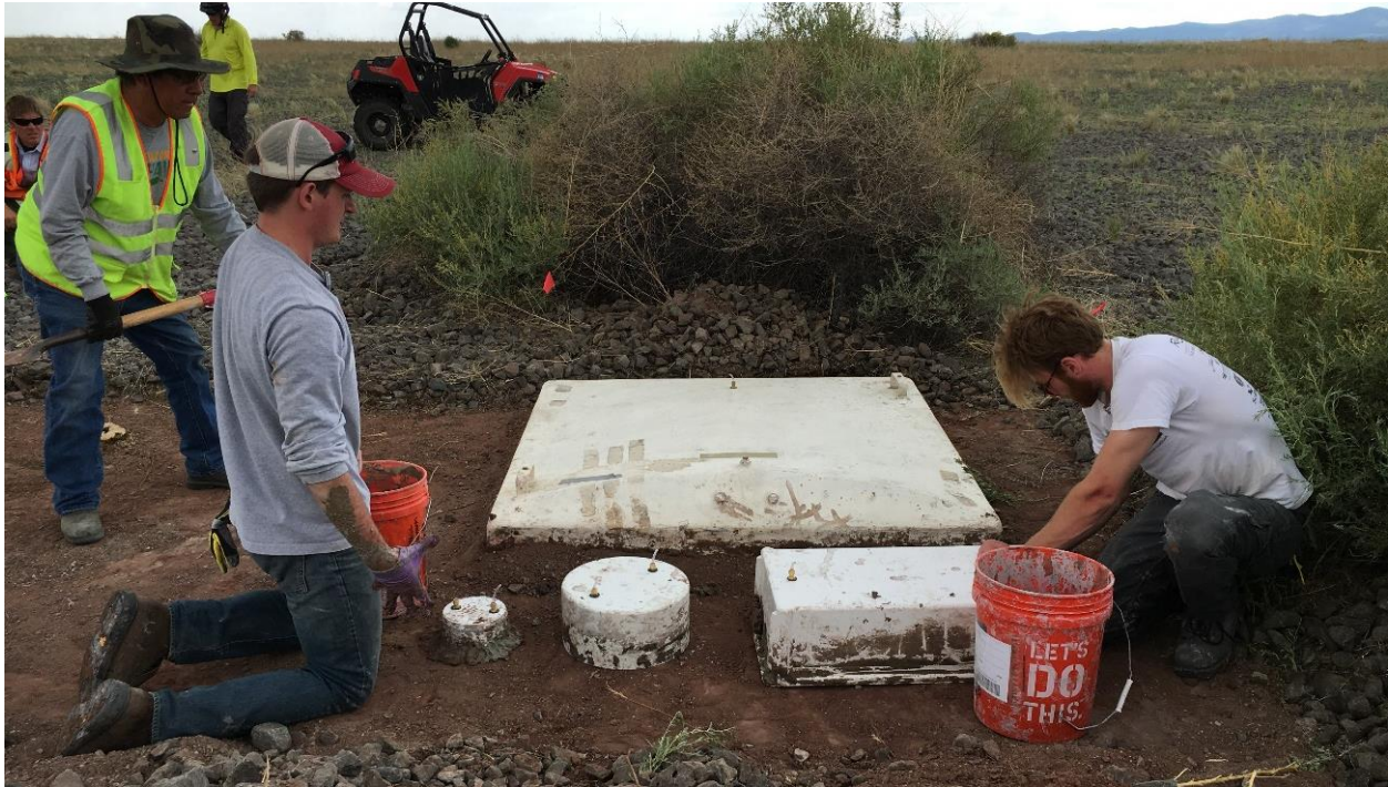
Figure 48 – Installation of flux chambers on the surface of the Rn barrier.
