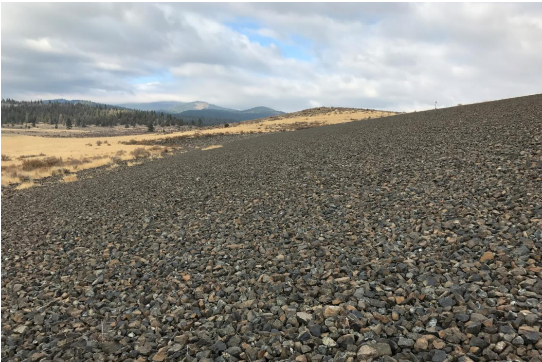
Figure 126 - Riprap covered slope of the disposal cell looking North.
