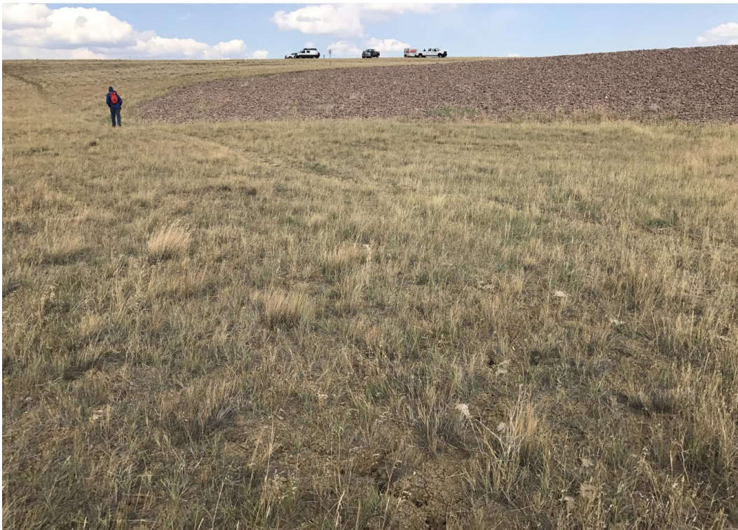
Figure 84 – Riprap on 5:1 slope looking North from lower deck.
