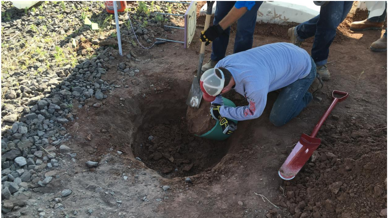
Figure 54 – Removal of a 350 mm diameter block sample from the Rn barrier.
