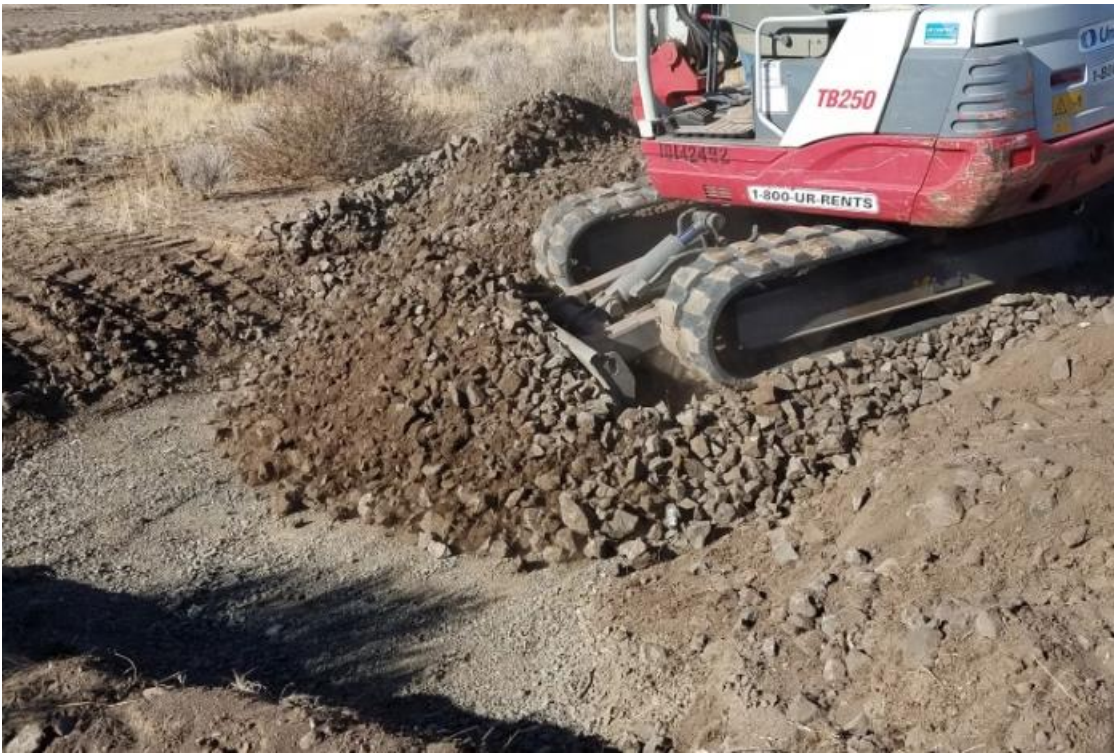
Figure 134 – Replacement of the protective layers using an excavator.
