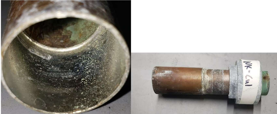
Figure A-60. Inside of a copper lateral obtained from Waukesha.
