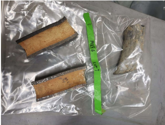
Figure A-12. Longitudinal cross section of a lead pipe harvested from Milwaukee. The tan color of the corrosion scale is characteristic of lead carbonate minerals.
