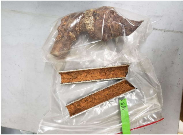
Figure A-55. Cross-section of a cast iron lateral obtained from Waukesha. Rounded tubercles and significant corrosion accumulation are noted.
