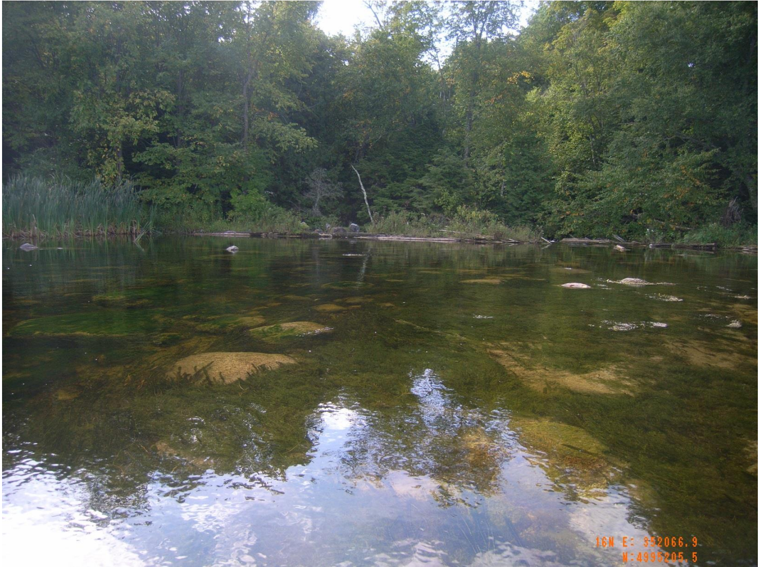
Figure 2. Upstream photograph of the Lake Dam located approximately two km downstream of the entrance into Upper Bass Lake on the West Branch of the Wolf River, Menominee Indian Reservation, Menominee County, Wisconsin.
