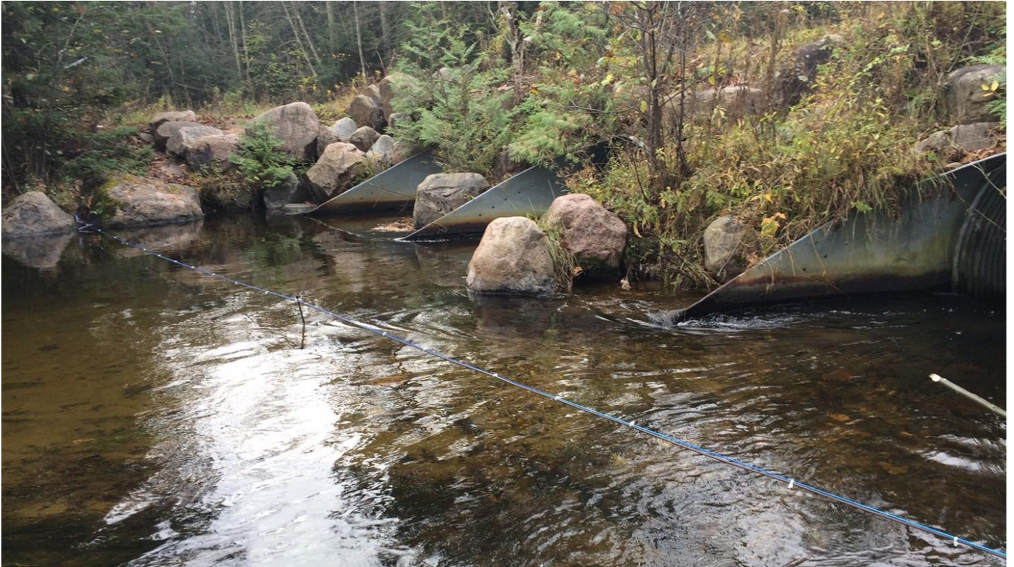
Figure 8. Culvert antenna (2U) positioned at the culvert complex on the West Branch of the Wolf River, Menominee Indian Reservation, Menominee County, Wisconsin. Antenna locations are shown on the map in Figure 6.
