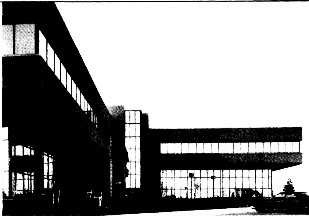
Headquarters Building, Automotive Operations, Troy, Michigan
