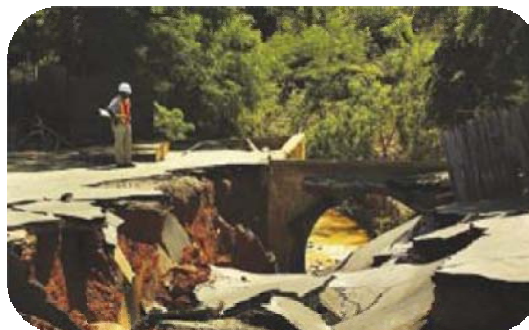
Figure 1.5: Failure of a 30 year old, 96" diameter CMP in Hickory, North Carolina
