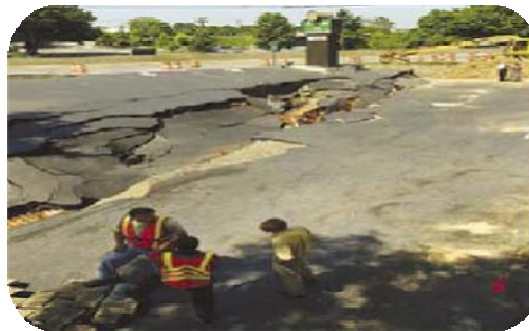
Figure 1.4: Failure of 126" diameter CMP in Charlotte, North Carolina
