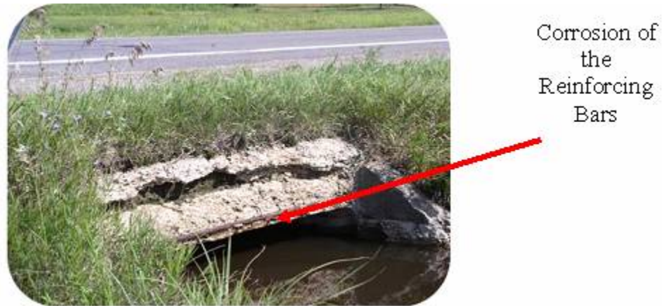
Figure 9.11: Condition of Culvert Structure 31000131B05
