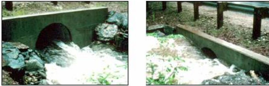
Figure 2.2: Culverts functioning as Inlet Control (Source: Hydrocad Storm Water Modeling, 2008)
