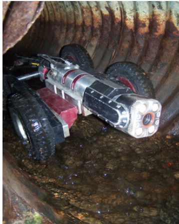
Figure A9.1: CCTV Camera in a Partially Flowing Culvert
