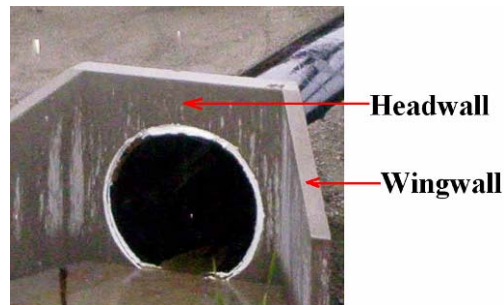
Figure 2.10: Culvert Showing Headwall and Wingwall
