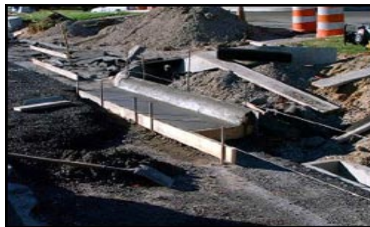
Concrete Paving of Earth Slopes
