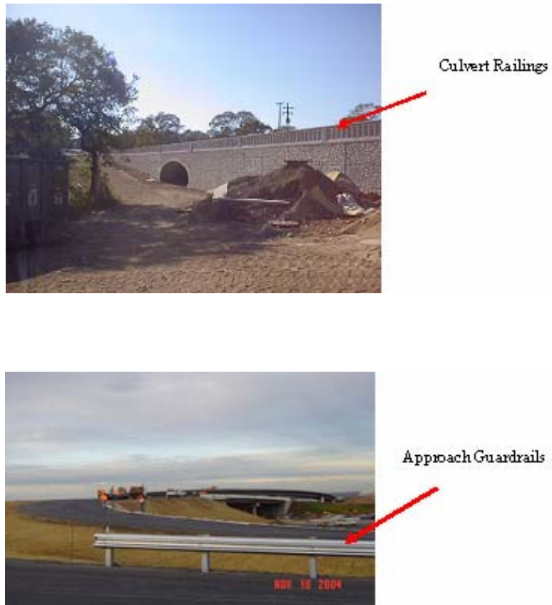
Figure A2.8: Safety Items for Culverts
