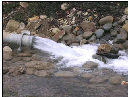
Figure 2.4: Culvert Flowing under Pressure Flow (Source: Eatonvillenews.net, 2008)
