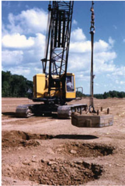
Figure 2.27: Dynamic compactor equipment, crane, and reinforced concrete falling weight (Source: TerraSystem 2011)
