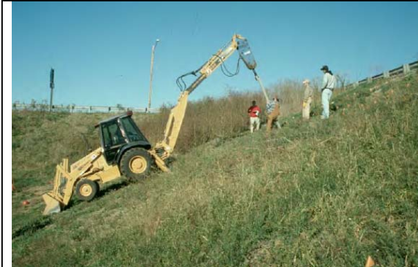
(a) Backhoe mounted hammer
