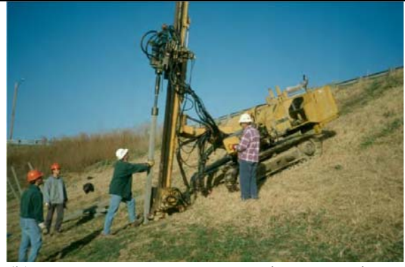
(b) Davey-Kent DK100B track-mounted hydraulic rig
