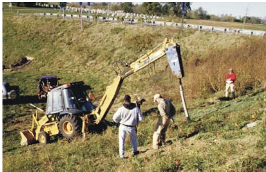
Figure 2.15: Installation of recycled plastic pins to stabilize surficial failures (after Loehr et al., 2000).
