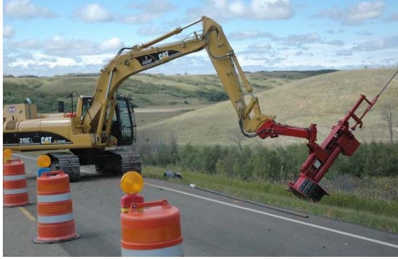
(a) Soil nail launcher
