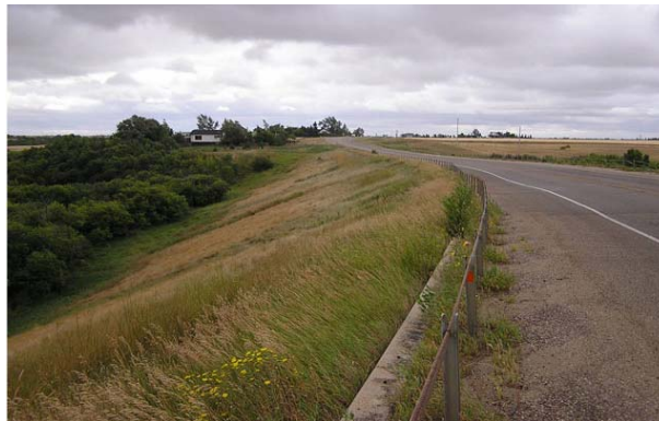
Figure 2.18: Highway 363 slope south of Moose Jaw, Saskatchewan, was stabilized with launched soil nails (SNL, 2007).
