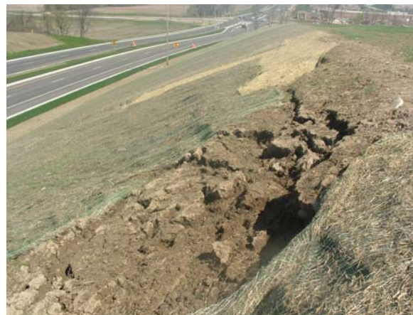
(c) Picture of the shallow slope failure
