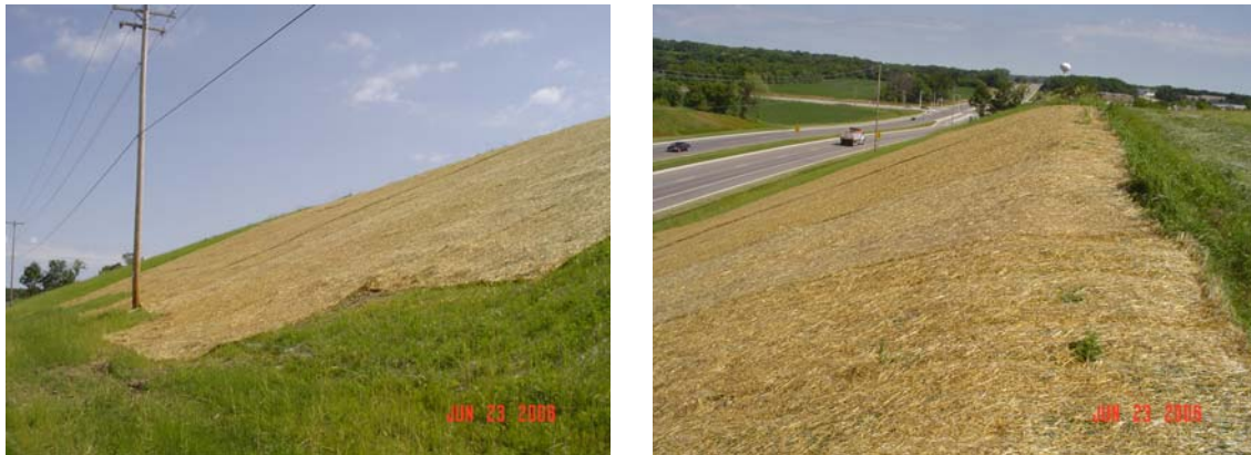
Figure 2.27: Pictures of the repaired shallow slope failure at STH-164.
