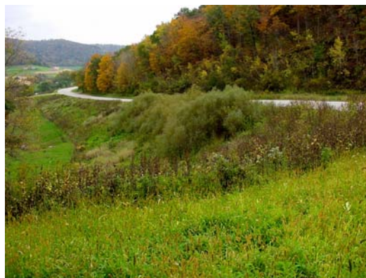
(b) Stabilized slope
