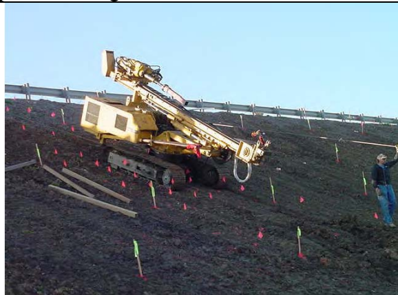
(e) Davey-Kent DK100B track-mounted hydraulic rig
