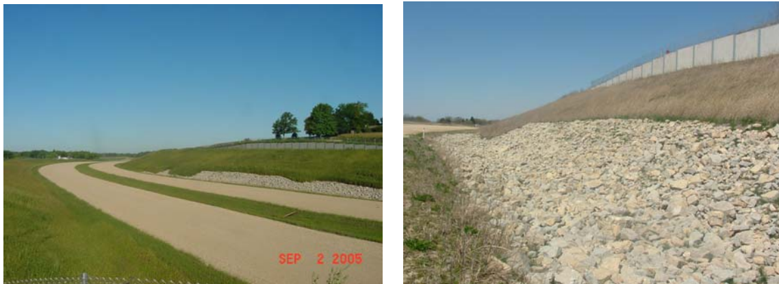
Figure 2.29: Riprap repair of shallow slope failure at STH-16.
