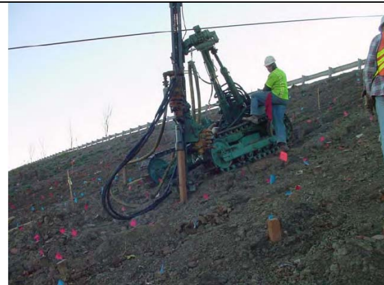
(f) Ingersoll Rand CM150 track-mounted pneumatic rig
