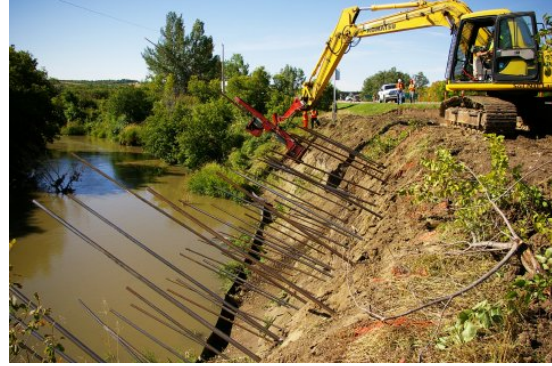
(b) Installation of launched soil nails
