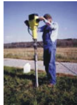
Figure 2.15: Installation of recycled plastic pins to stabilize surficial failures (after Loehr et al., 2000).
